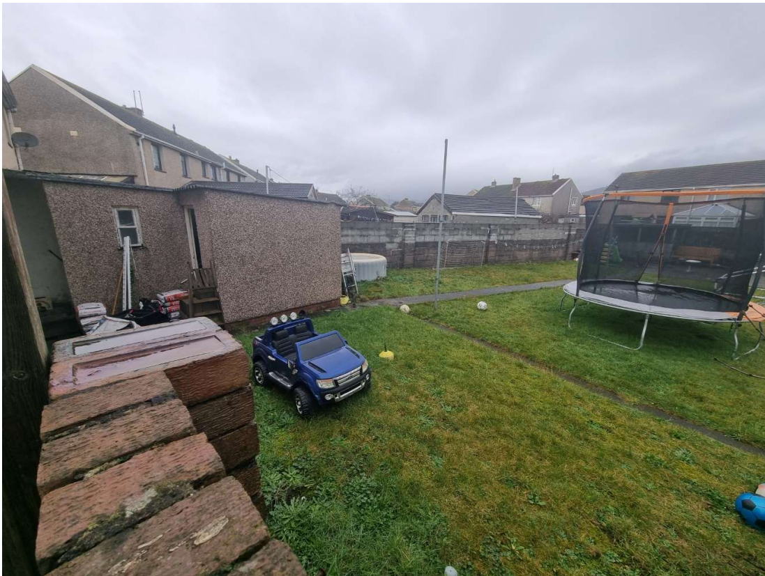
View of large rear garden area with current outbuildings/rear extension area
