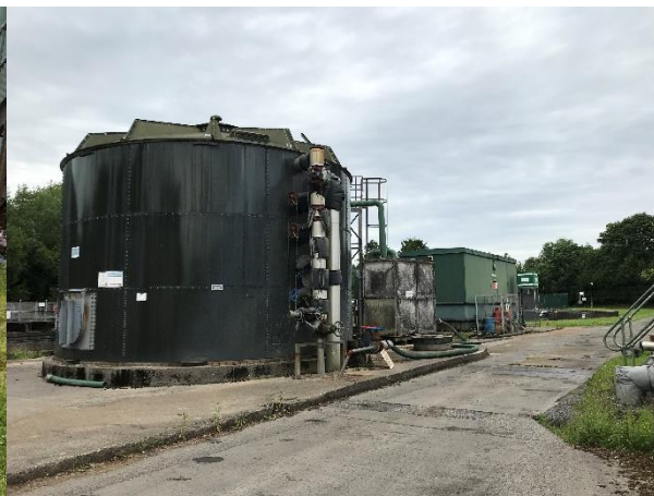
Photograph 2: Hardstanding and built structures associated with the WwTW.
