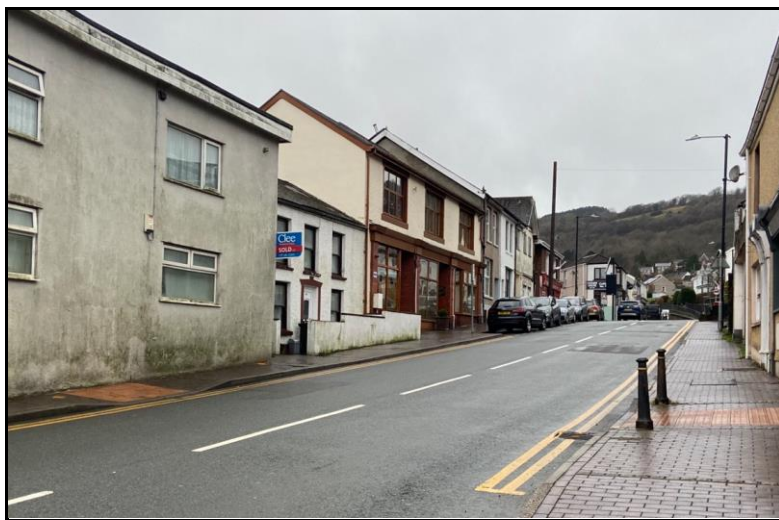
Photograph 1 – Showing Double Yellow Lines Adjoining the Property and the Dedicated Parking Bay to the South of the Site
