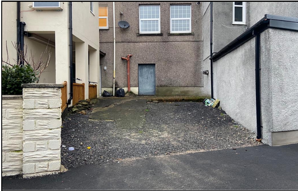
Photograph 5 – Further Illustrating Parking Arrangements in Rear Lane for Neighbouring Properties.
