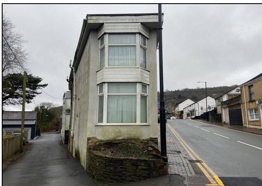
Photograph 2 – View of the Eastern Side of the Building
