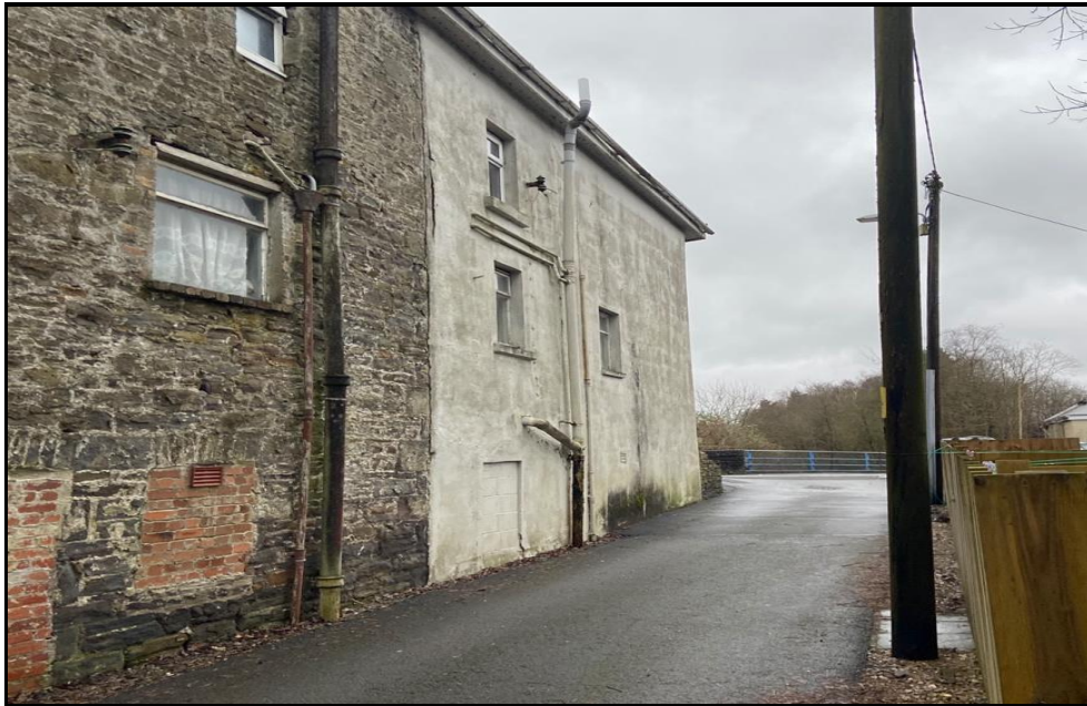
Photograph 3 – Showing the Rear Lane
