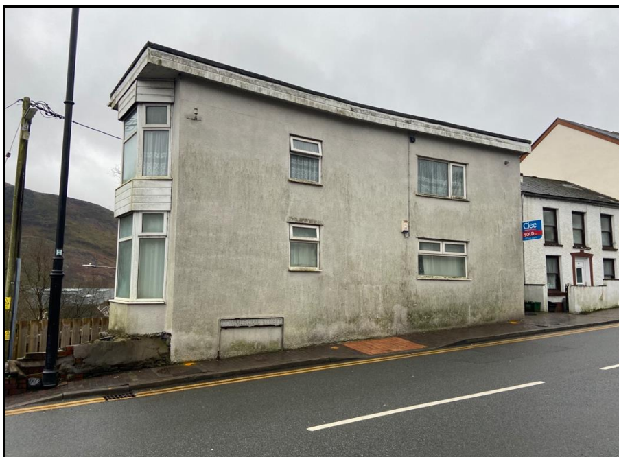
Photograph 1 – Existing Building Viewed from Commercial Street
