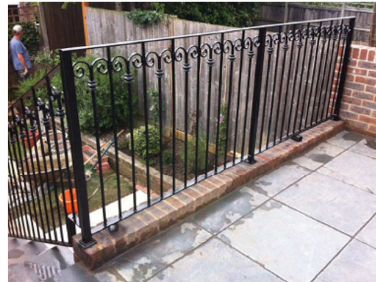
Example of Guardrail - galvanised steel and in-line bars- painted black
