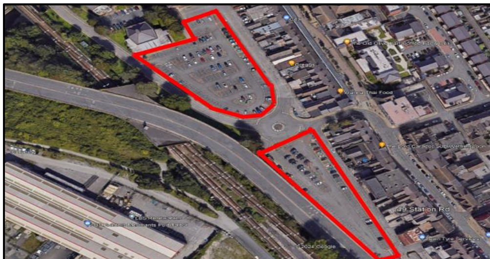
Photograph 5 – 87 Station Road Car Park to the South and Bethany Square Car Park to the North
