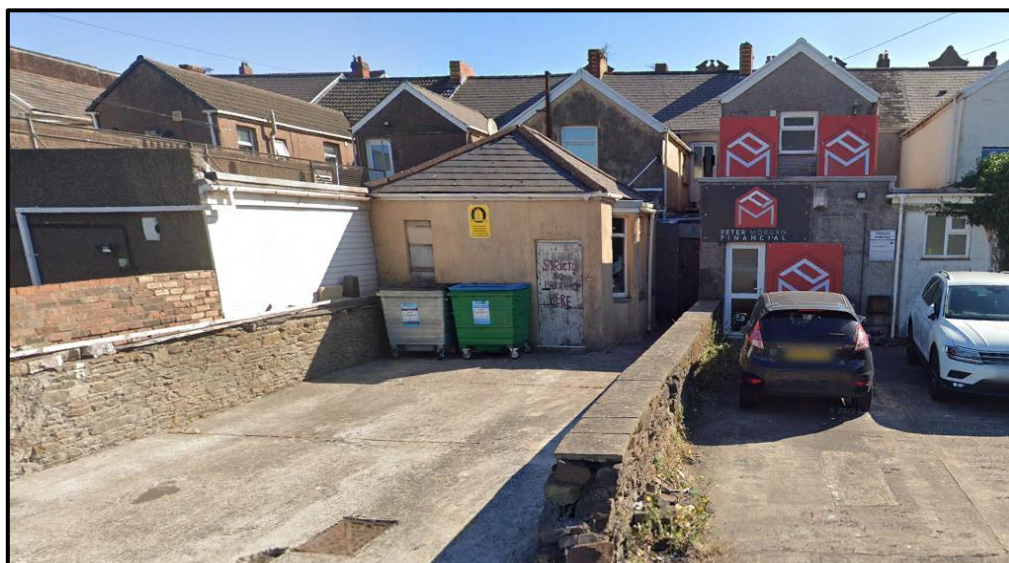
Photograph 2 – The Rear of 49 and 51 Station Road
