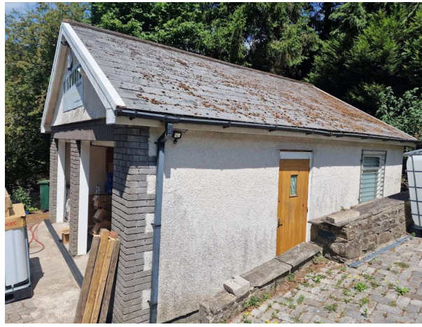
Figure 9: Existing garage at Windways – 50 Afan Road
