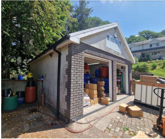
Figure 8: Existing garage at Windways – 50 Afan Road
