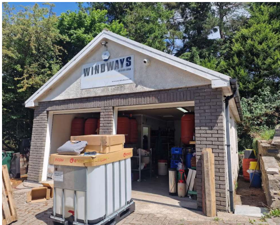
Figure 10: Existing garage at Windways – 50 Afan Road
