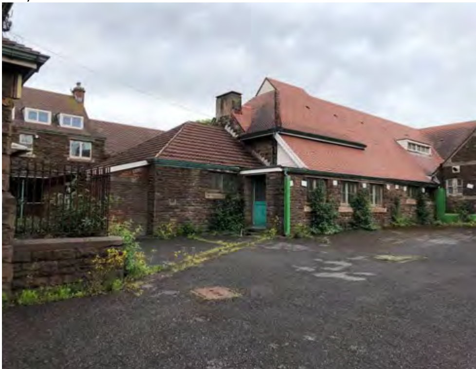
Photograph 5: View of central and northern structures located along York Place, facing north-east.
