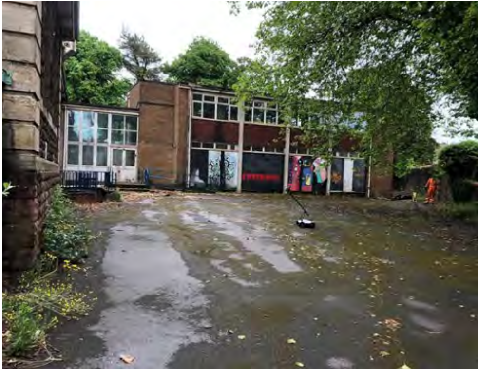
Photograph 7: View of structures within the south-eastern corner of the site, with partial basement, facing south-east.
