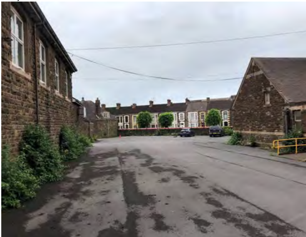
Photograph 3: View of existing structures and hardstanding, taken from the north-western corner of the site, facing south towards Devonshire Place.
