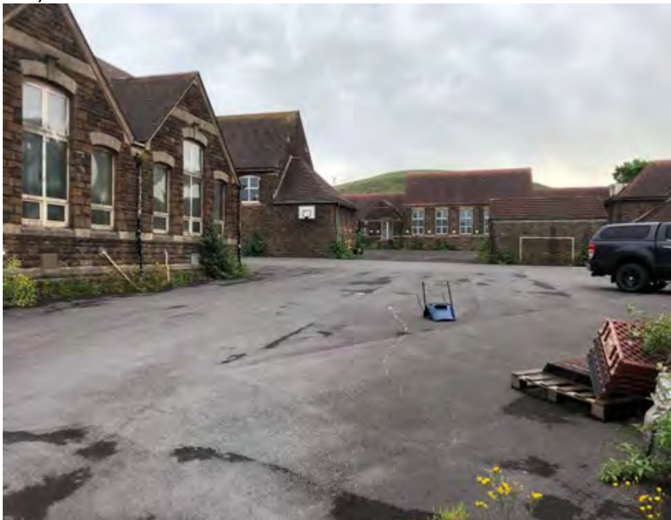
Photograph 1: View of site and existing structures from entrance gate, facing east.
