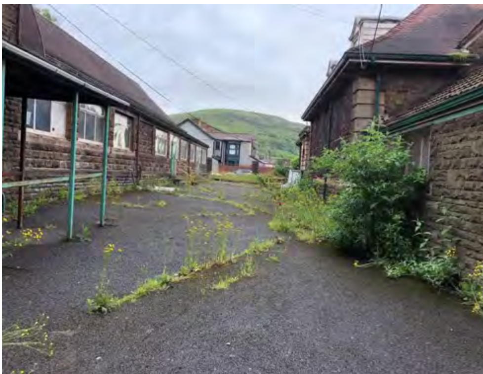
Photograph 6: View of structures located within the north-eastern area of the site, facing east towards Talcennau Road.
