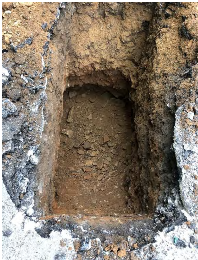
Photograph 4: View of TP01.
