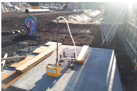
H14 adjacent to digging hole
