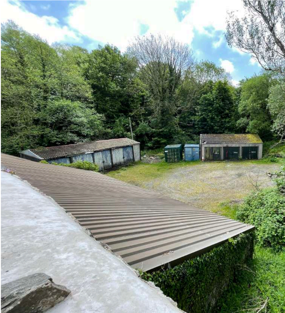
Existing facilities buildings and storage containers to the pump house service yard.
