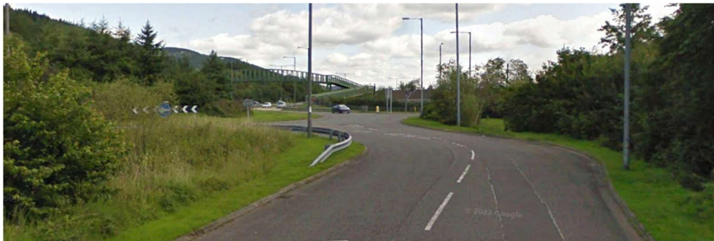
Access Road connecting to the A465 and the B4434.
