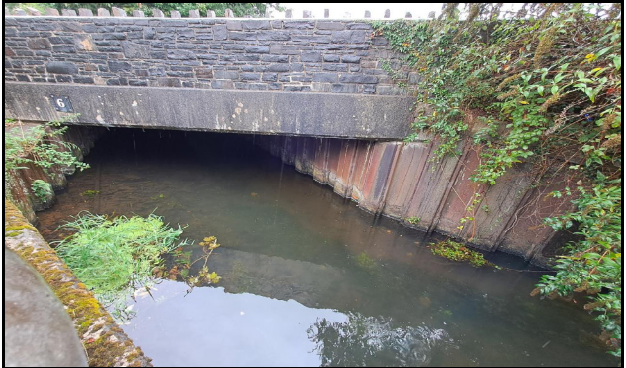
Plate 4 – Bridge in the north west corner from the site (Holly Street Bridge).
