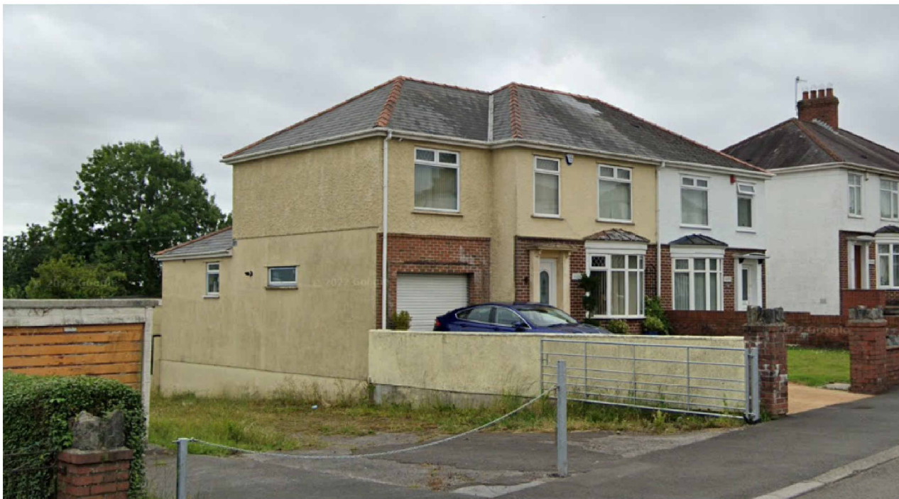
Existing Extension at Neighbouring Property (57 Crymlyn Road)
