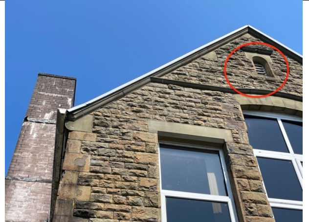
Another estimated location is the louvered window on south side pitched roof, chimney of boiler room can be seen in photo
