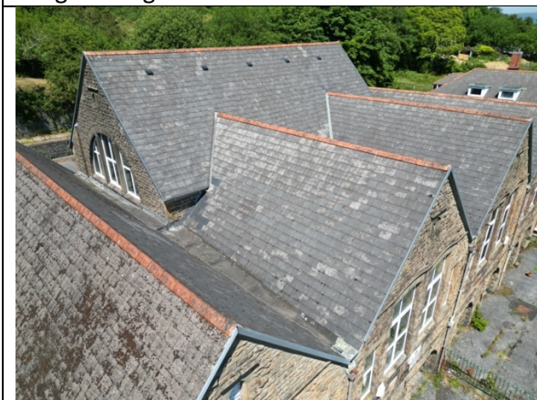
Roof structure juniors school
