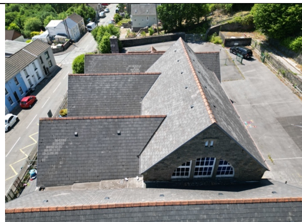
Roof structure juniors school
