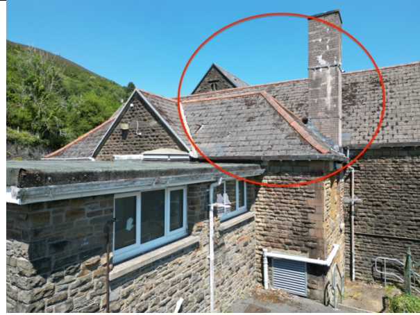
Estimated area of emergence above boiler room
