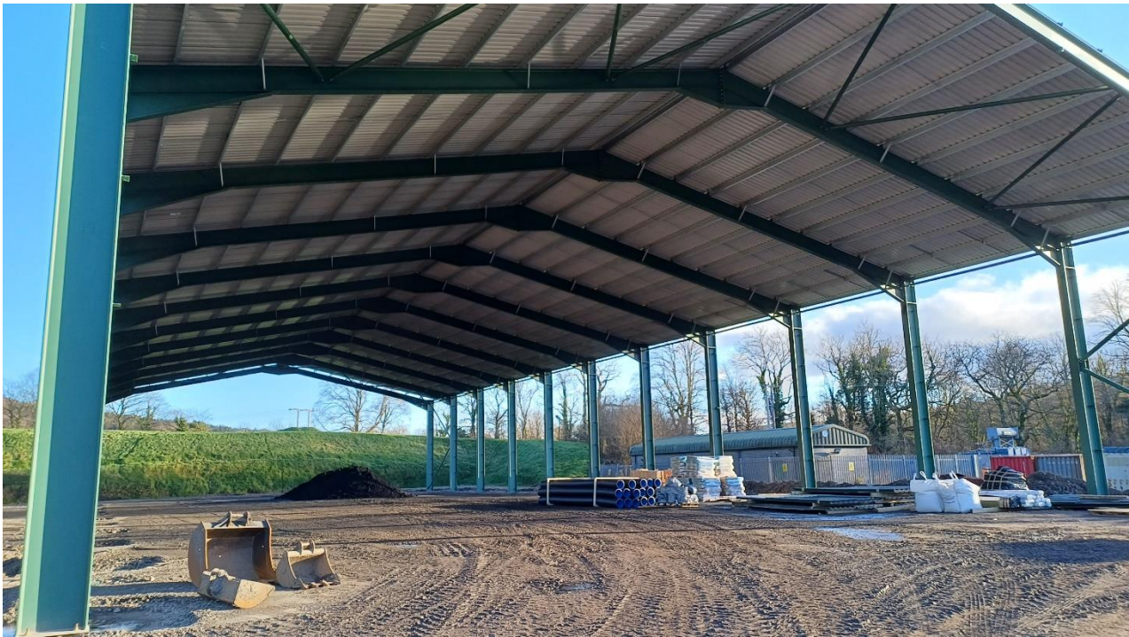
Picture Taken: 10/01/2024 Photograph No. 2 Title: View of the digger buckets and various materials temporarily stored on the southwestern half of the site.
