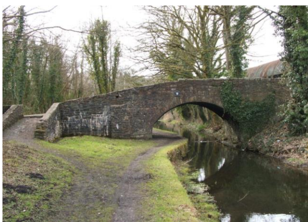
Figure 1 Ynysmeudwy Uchaf Bridge - north elevation
