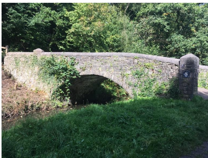
Figure 1 Ynysmeudwy Ganol Bridge, viewed from the south
