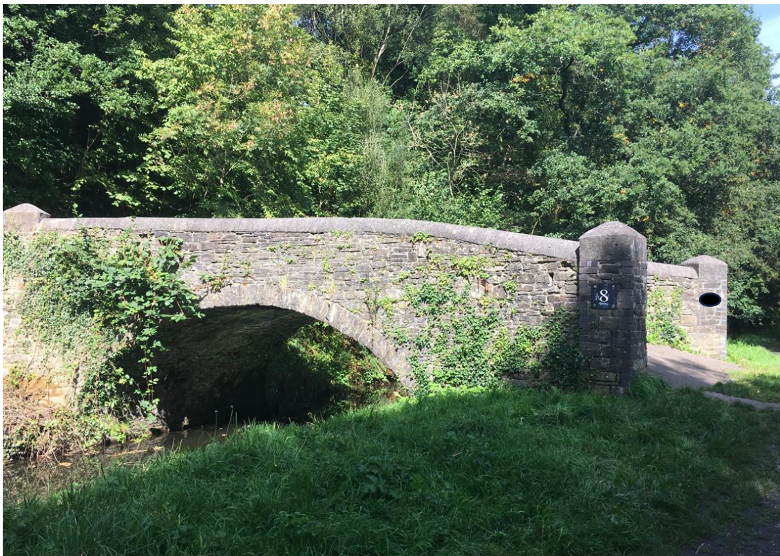
View towards south elevation with proposed location of plaque. Vegetation and repointing to be addressed (as previously agreed) during a heritage skills week in March 2024
