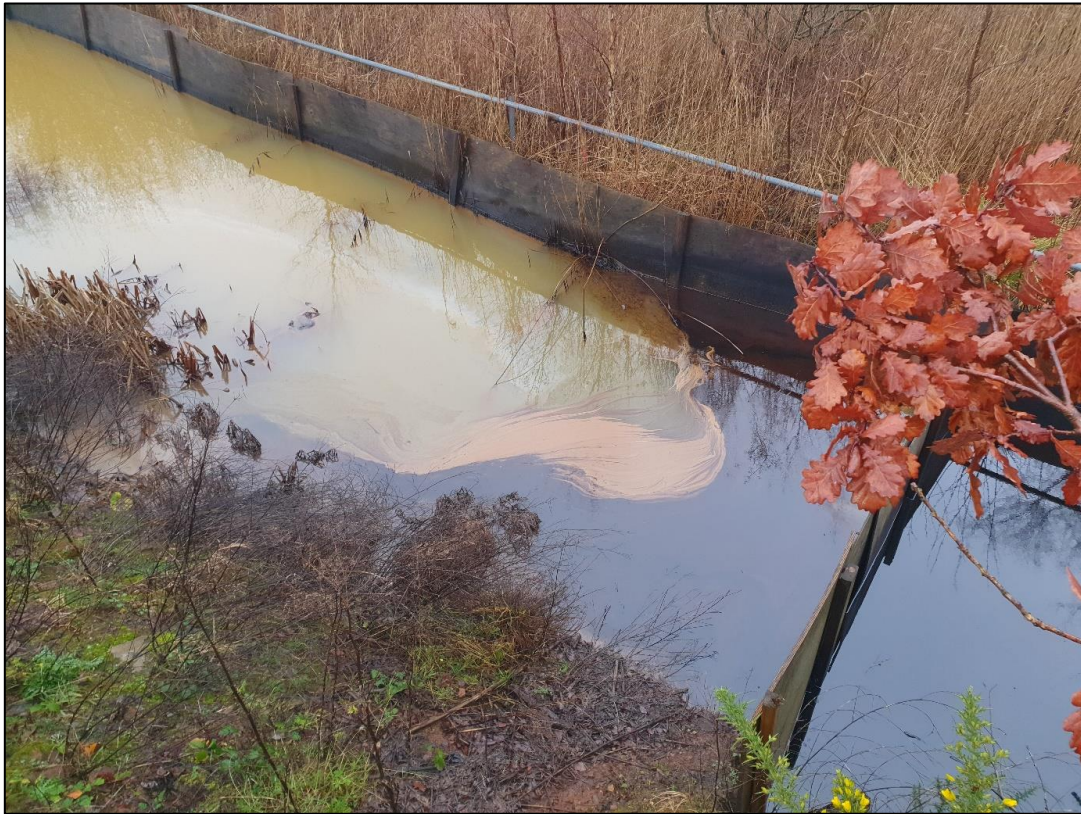
Figure 13: Hydrocarbon contamination visible in surface water ditch on northern perimeter of the site (December 2022).
