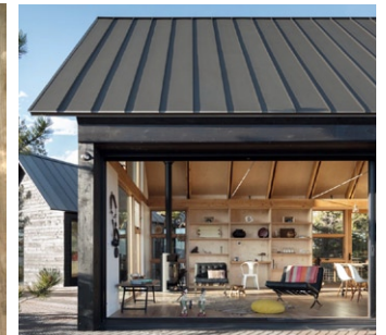
Slate grey standing seam roof
