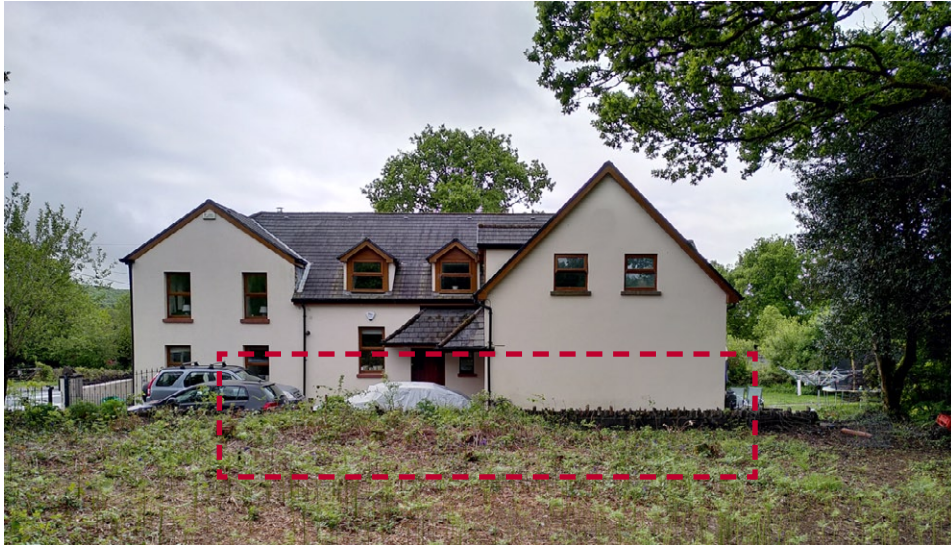
View from the top of the site
