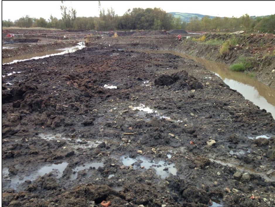
Photograph 4: Peat at base of excavation in northern part of Zone 2
