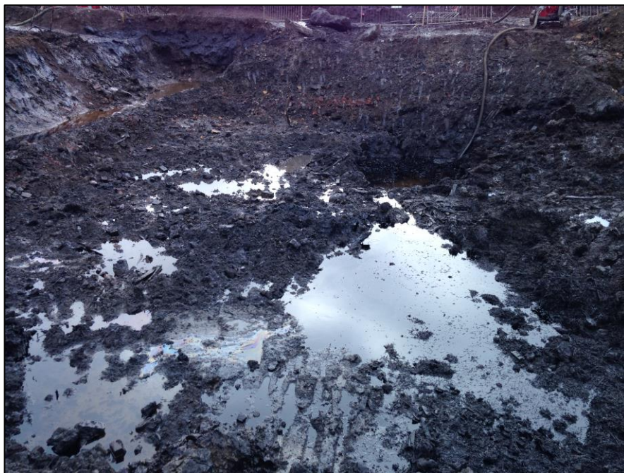
Photograph 7: Oil Recovery from the excavation in Zone 3
