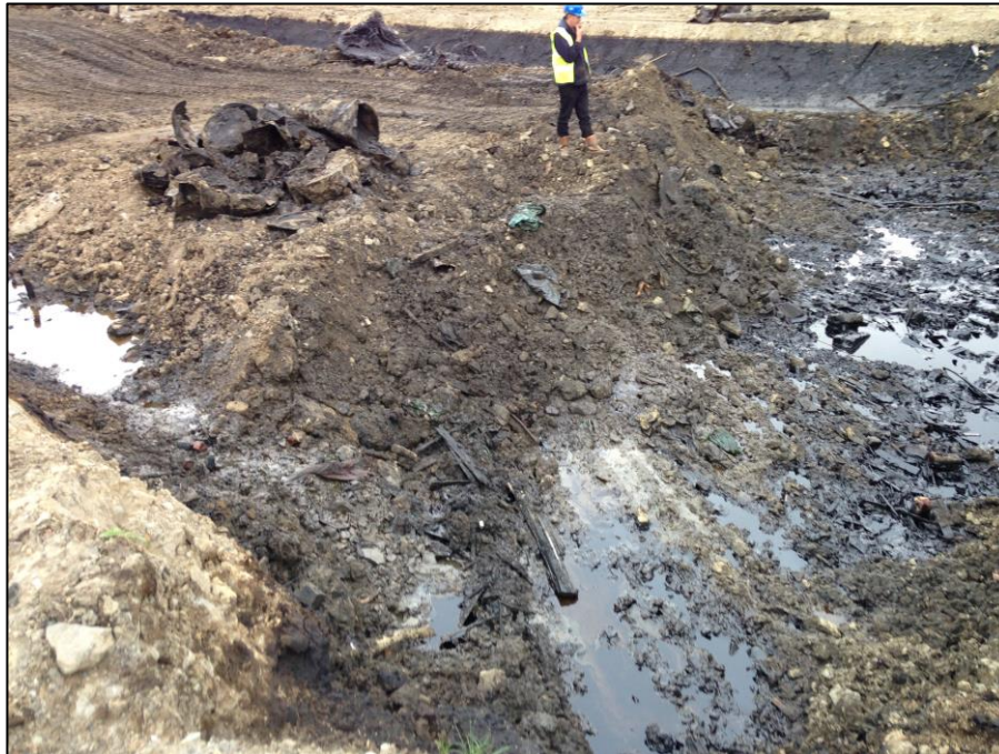
Photograph 6: Base of excavation and partial backfilling in the southern part of Zone 2
