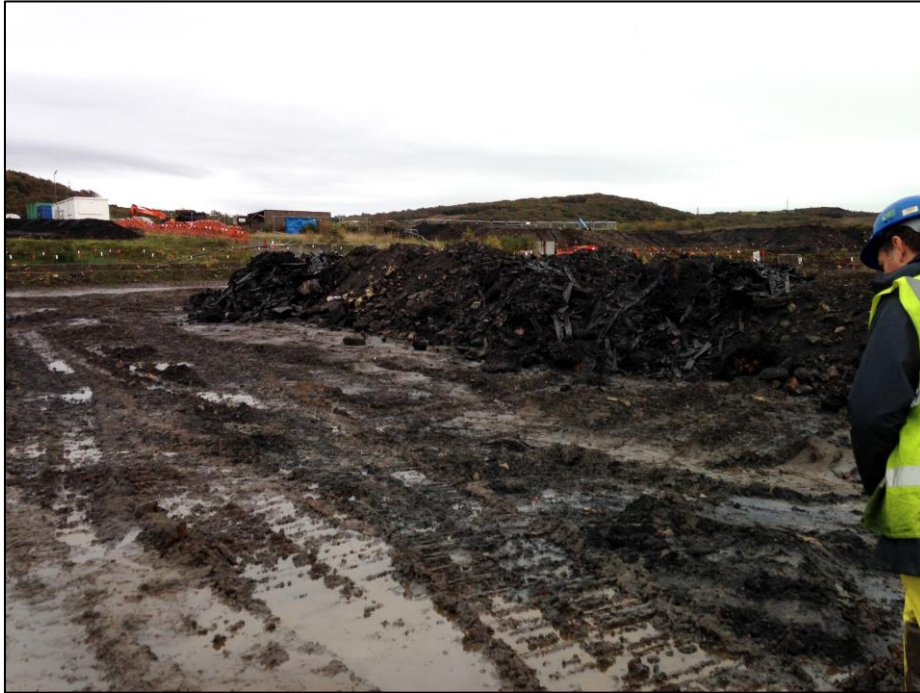
Photograph 8: Arisings from excavations
