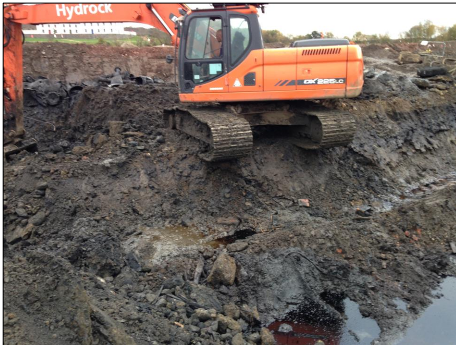
Photograph 5: Excavation of waste deposits in Zone 2
