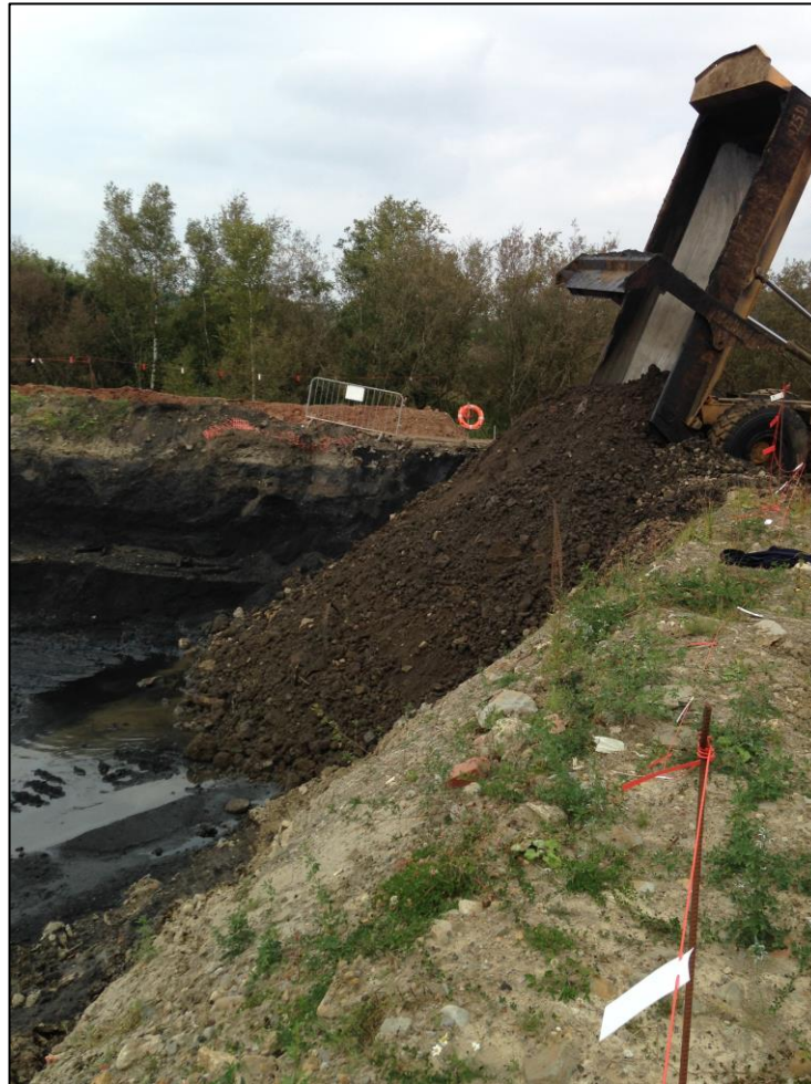
Photograph 3: Backfilling of drained soils into Zone 1 (north east corner)
