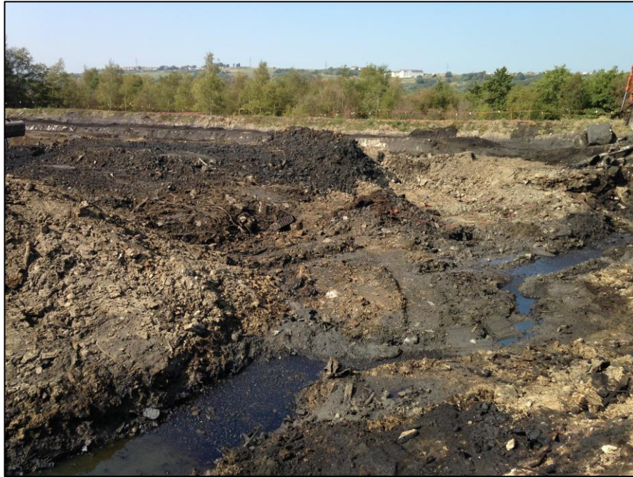
Photograph 1: Excavation in Zone 1
