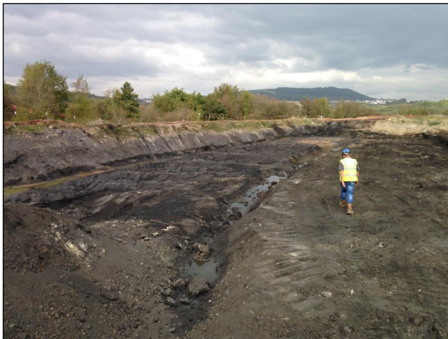
Photograph 2: Base of Excavation North of Zone 1
