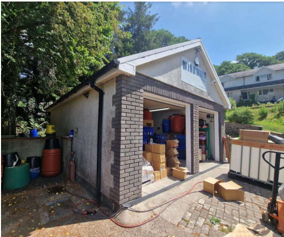
Figure 8: Existing garage at Windways – 50 Afan Road
