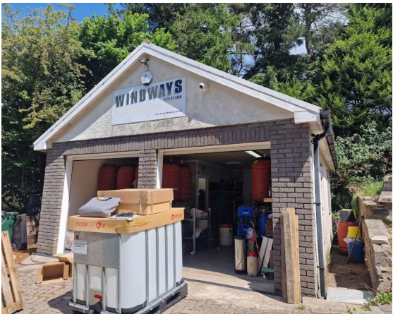
Figure 10: Existing garage at Windways – 50 Afan Road
