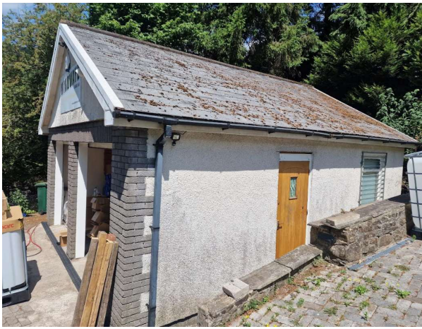
Figure 9: Existing garage at Windways – 50 Afan Road
