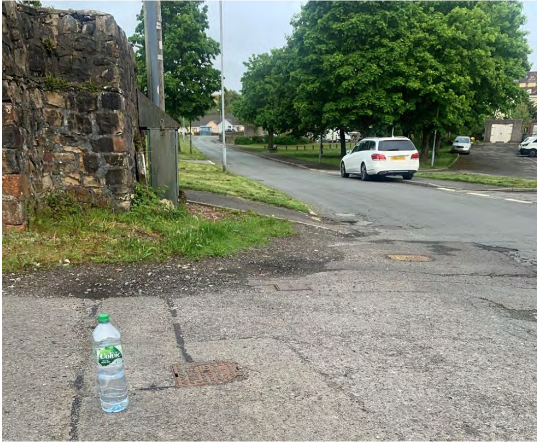
Plate 3.1 Visibility splay looking left from lane access
