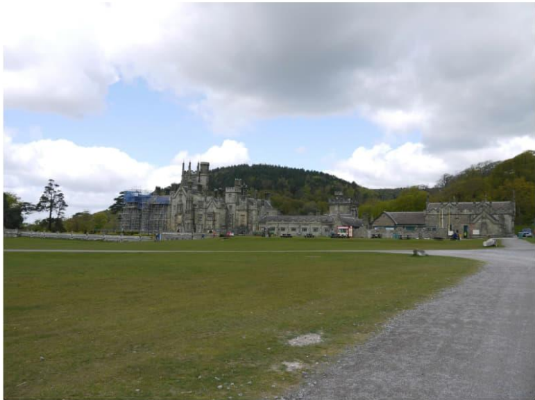
Photo 9: Margam Castle (LB 14170) and Service Buildings including Courtyard Walls at Margam Castle (23278) looking northwest
