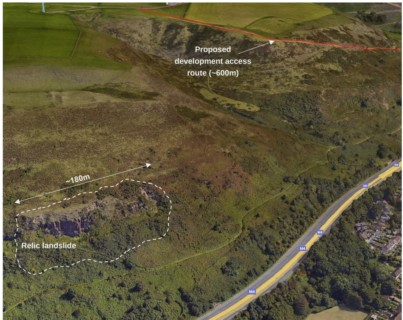
E2: Historic landslide southwest of the proposed development's access route. Google Earth Satellite imagery from 2021
