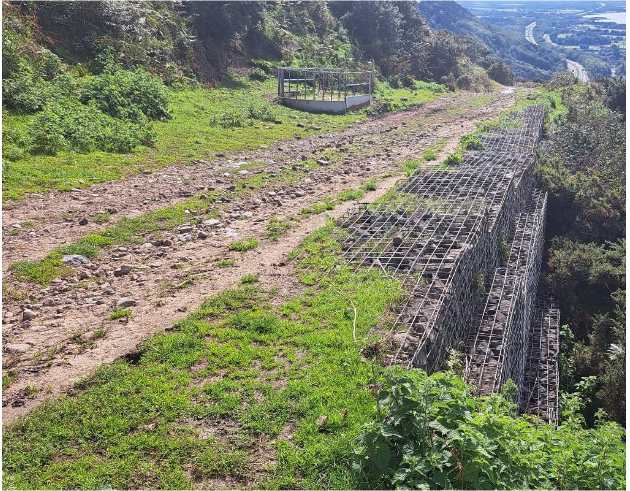
Figure A8: A pre-existing construction install to increase slope stability beside the access track (gabion baskets) located on the lower slopes of the current access track (278672E, 188030N)
