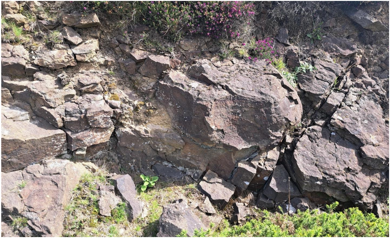
Figure A6: Sandstone (Rhondda Member) outcrop along the access track (278583E, 188196N) exhibiting an approximately 45-degree fracture plane (dotted yellow line). This outcrop is located on shallower-dipping ground along the current track compared to where the landslide deposits were observed which may explain why there hasn't been clear rock sliding/ground movement here
