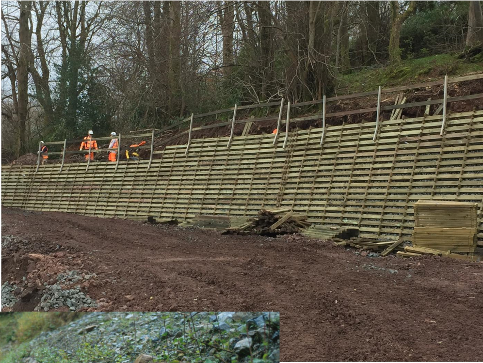
Figure G3: Example Crib Retaining Wall Options (ref: LaRiMIT & Phi Group)
