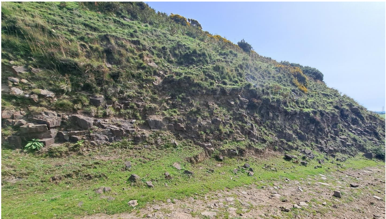
Figure A7: Sandstone (Rhondda Member) outcropping steeply beside the access track running northwest-southeast.
