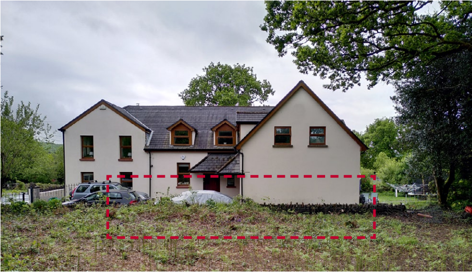
View from the top of the site
