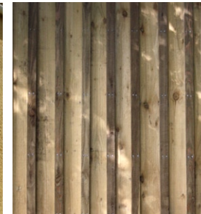
Timber cladding to workshop
