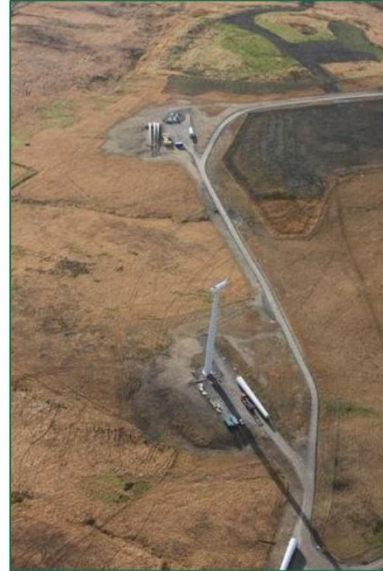
Photo: ESB's Mynydd y Betws wind farm under construction
