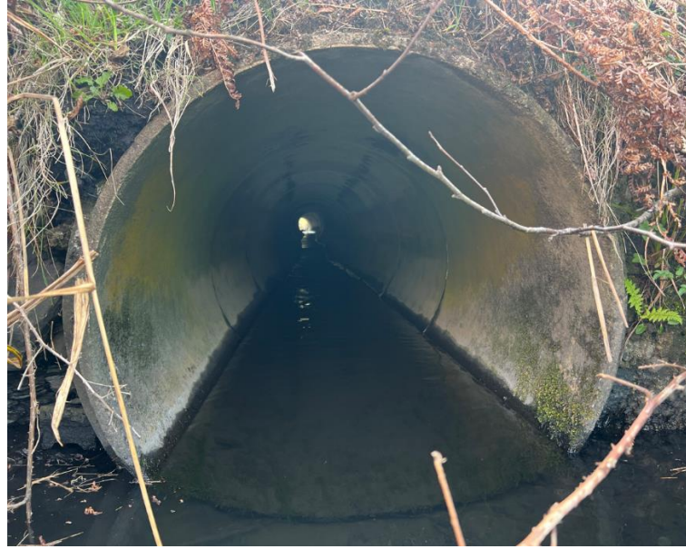
Figure 3: Picture of existing culvert
