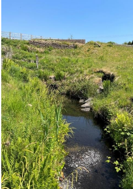
Figure 2: Picture downstream of the culvert
