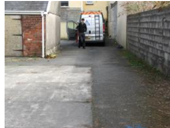
6: Neighbouring property built-up alongside boundary acting as wall
