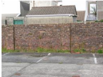
3: Side and rear brick wall (2100mm tall)
