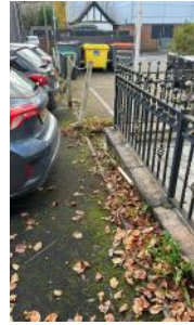
2: Front boundary with chain and side railings (1100mm tall)
