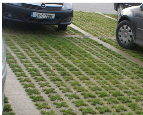
Figure 4: Grasscrete used and accepted widely for vehicle parking and as a surface drainage system
