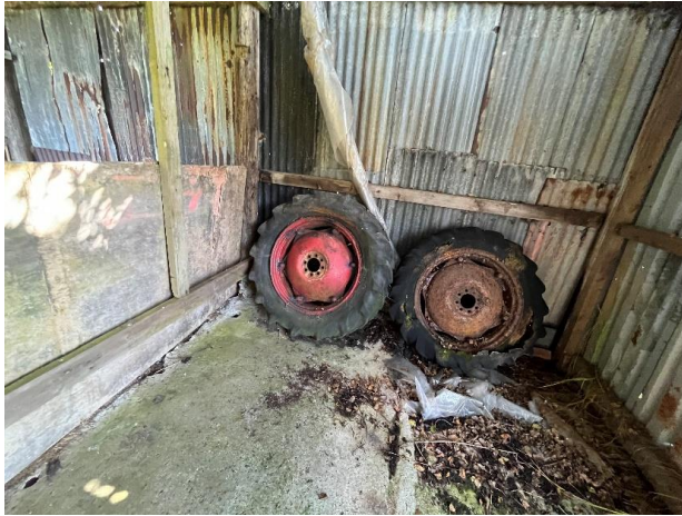
Tractor tyres on concrete floor – confirming agricultural related use
