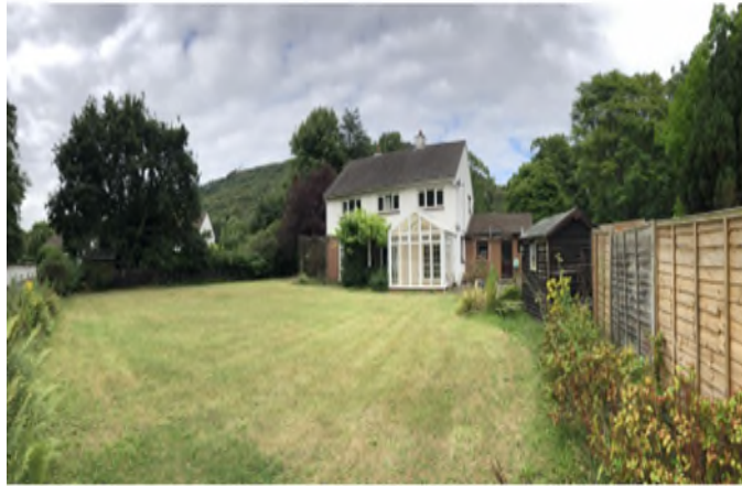
Image 1: Existing single family dwellinghouse
