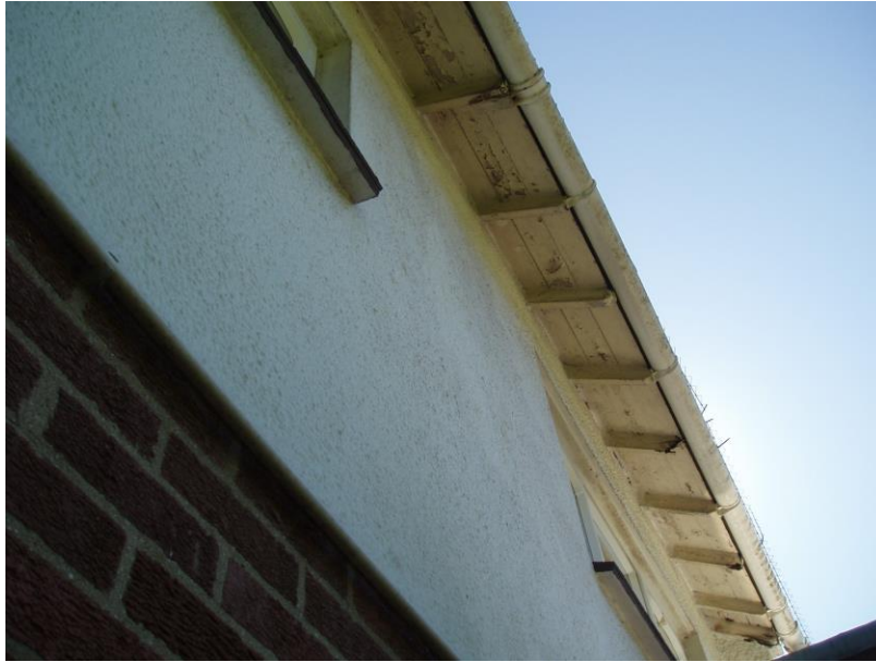
Both eaves and verges generally tight against bat entry.
