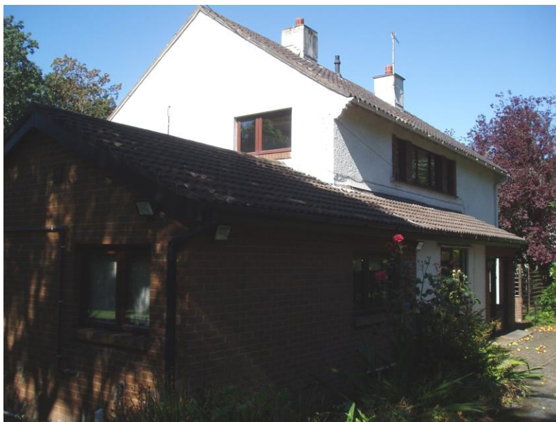
Southern gable and eastern elevation
