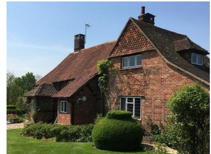
Figure 30: Hanging tiles and Catslip roof
