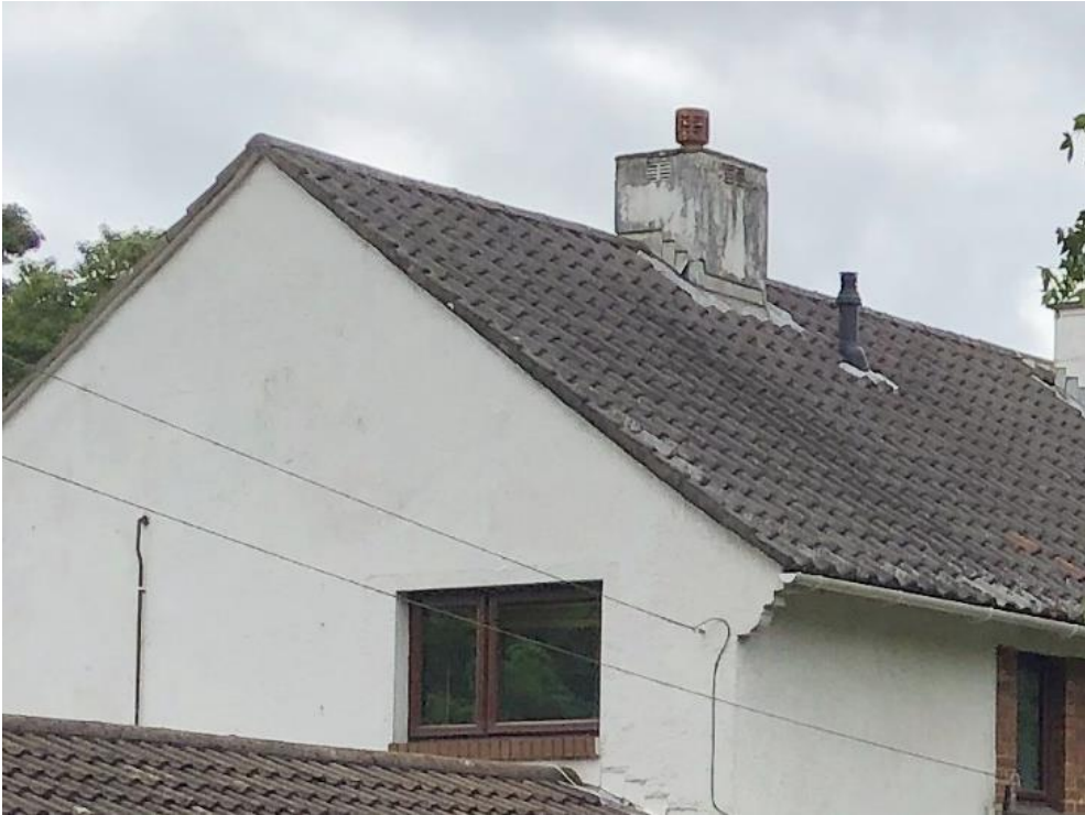
Figures 8 & 8.1: View from main pedestrian entrance & detail of render failing on chimneys
