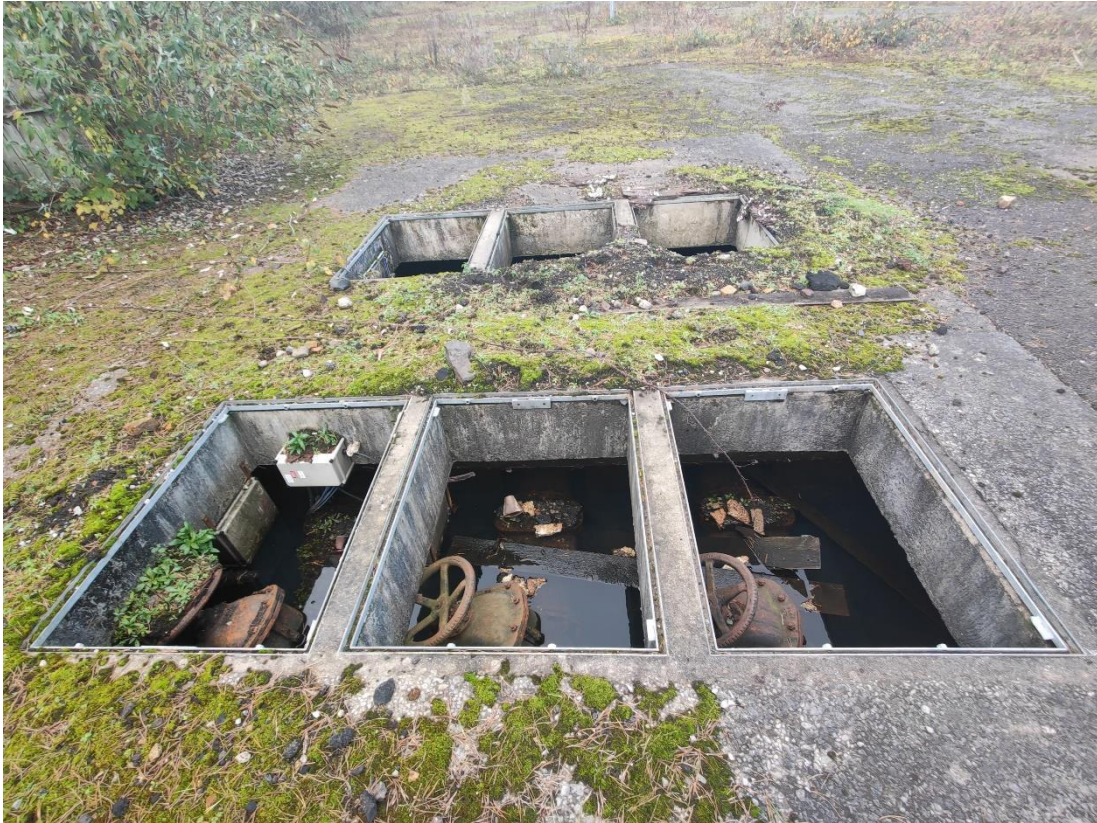
Plate 5: Disused drainage at the southern end of the site.
