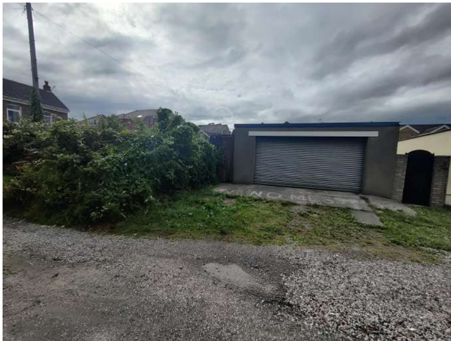
View of south hedge and neighbour garage from private access lane to south
