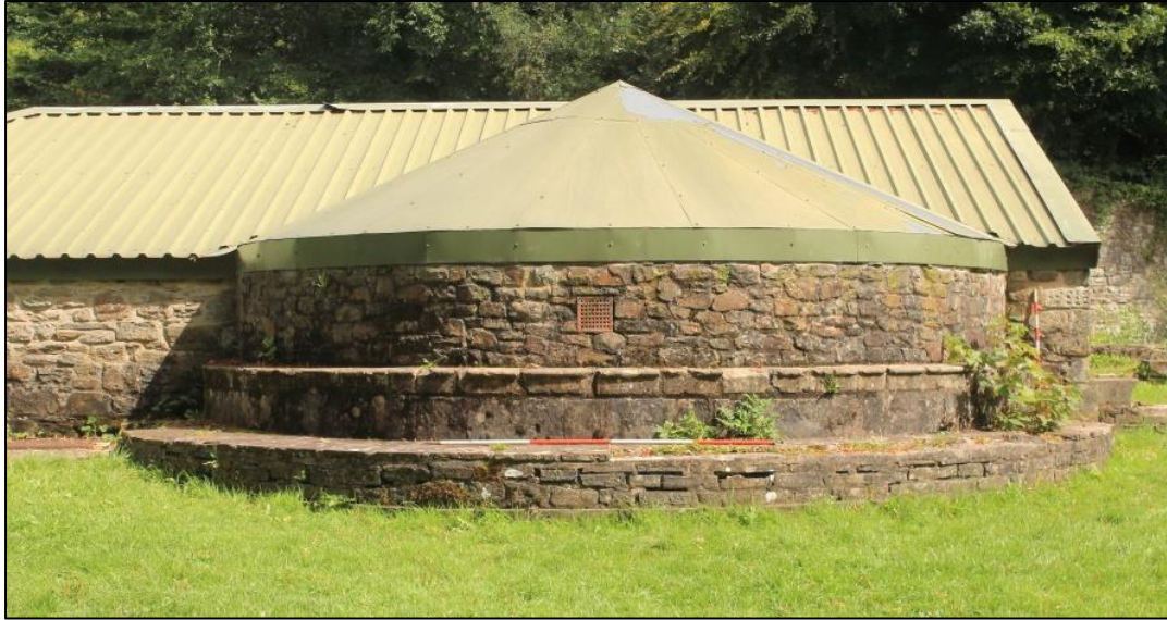
Photo 48: View east of the curved bay/tower base of the former drawing room. 2m scale.
