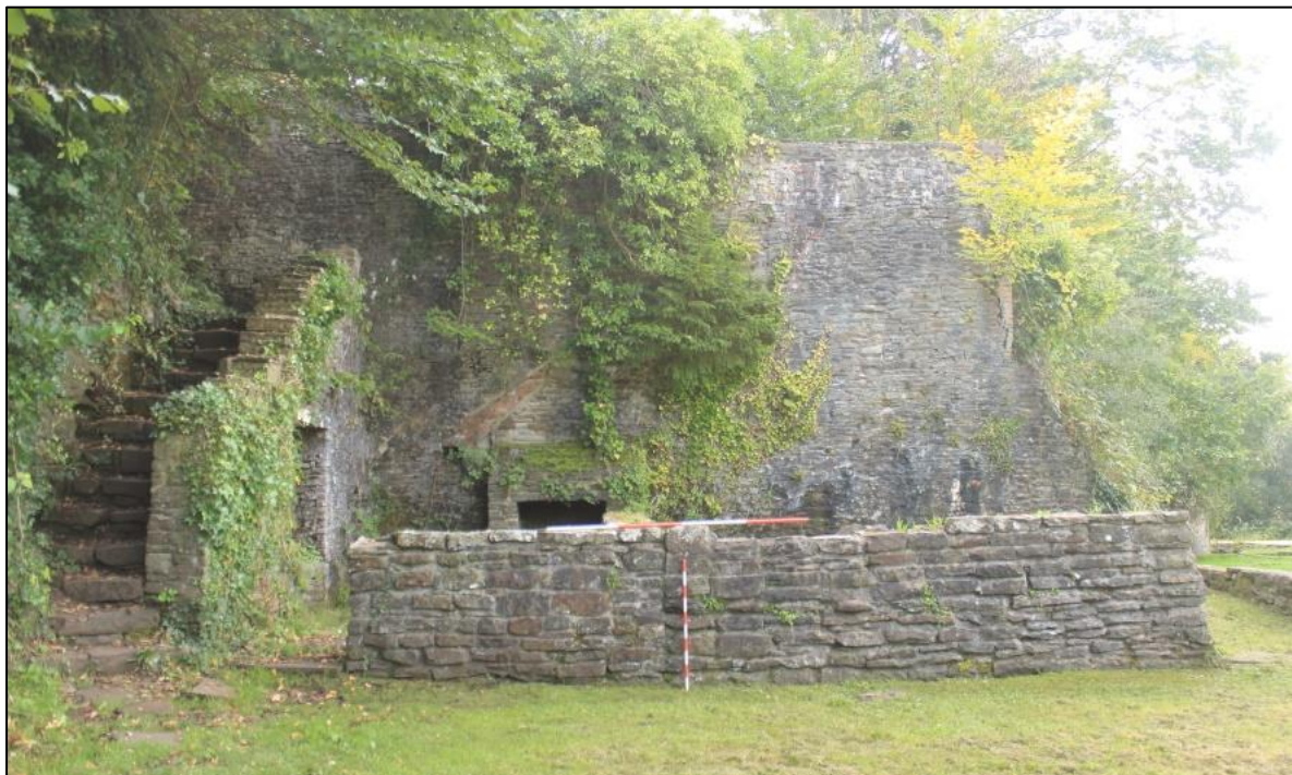
Photo 63: View south of the north and south walls of a former coach house and washhouse, with steps to a viewing platform above. 2m and 1m scales.
