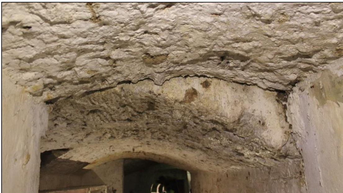
Photo 13: View north, detail of roof alignments at the entranceway between Room 2 and Corridor 1.
