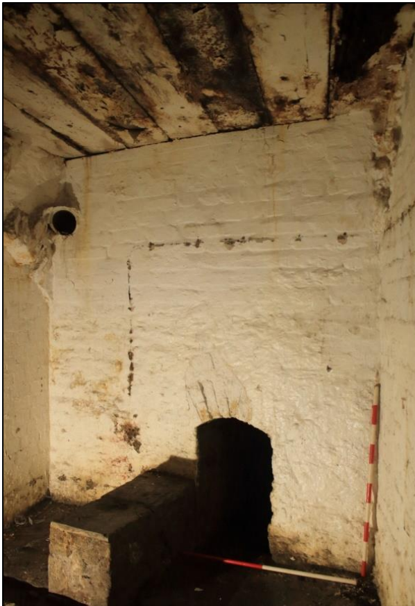
Photo 22: View west of the opening in the west wall of Room 4 (Compartment B). 1m scales.
