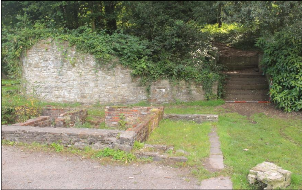
Photo 60: View east showing the stairs and retaining wall to the southeast of the house. 2m scale.
