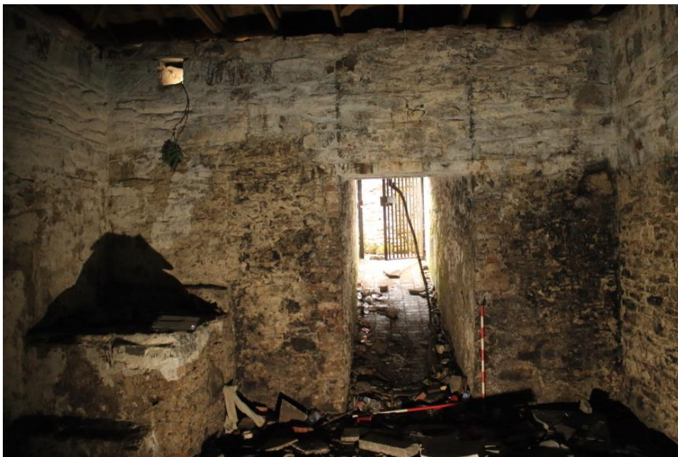
Photo 8: View east, Cellar Entrance to Room 2. 1m scales.
