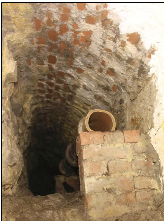
Photo 30: View north of pipework running to the rear of the eastern wall of Room 4, opening into the western end of Corridor 3.
