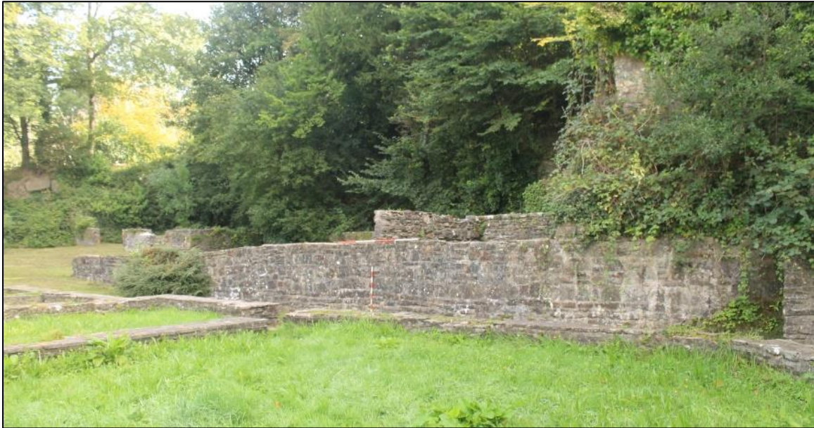
Photo 62: View northeast of retaining wall along the eastern side of Gnoll House. 2m and 1n scales.
