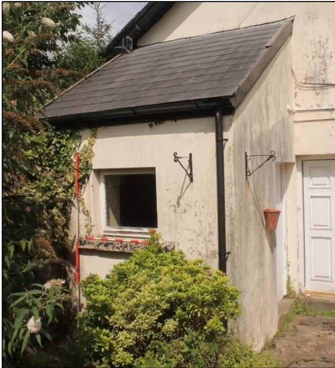
Photo 93: View northwest of the rear lean-to attachment.
