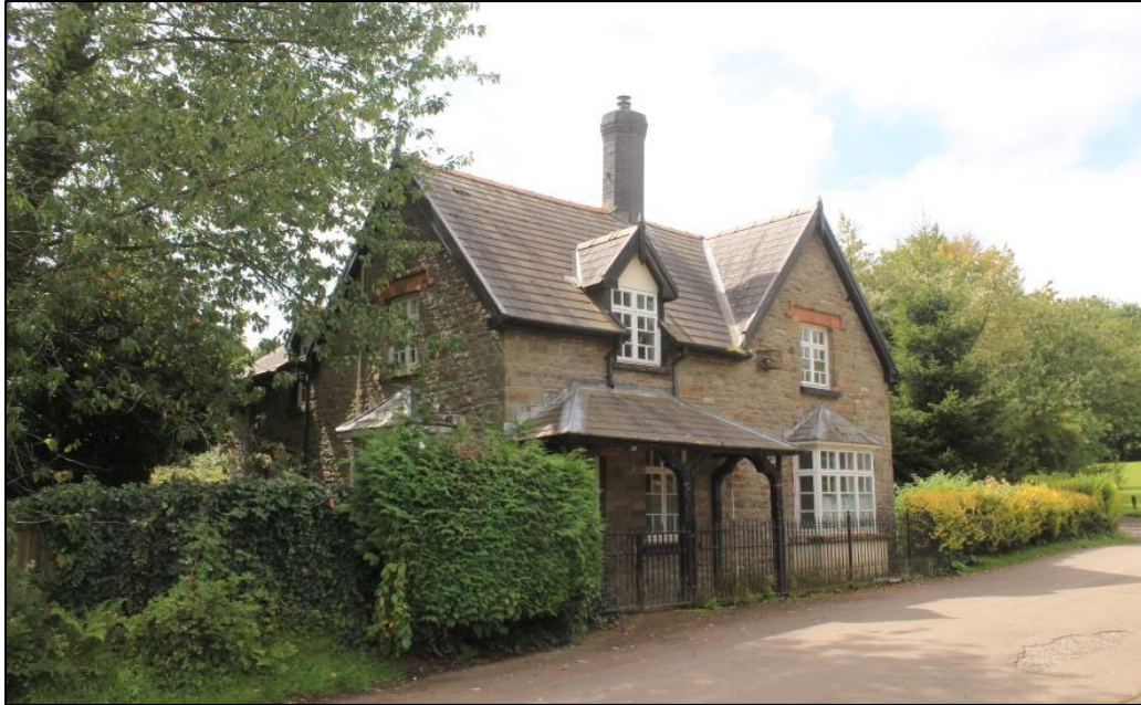
Photo 81: View southwest showing the front elevation of Pond Cottage.
