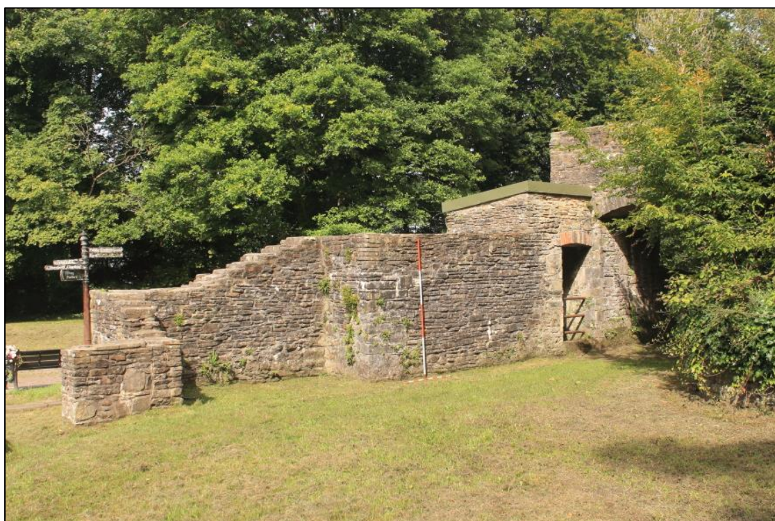
Photo 80: View west showing the wall on the south side of the entranceway structure. 2m scale.
