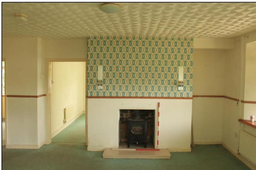
Photo 102: View west of living room fireplace. 1m scales.
