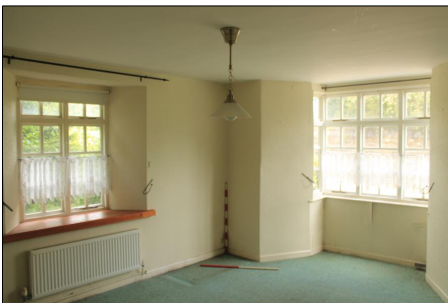
Photo 104: View northwest. Ground floor parlour/bedroom. 1m scales.
