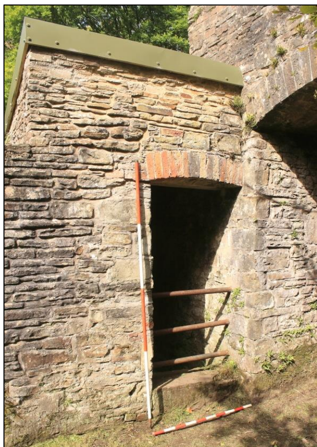
Photo 78: View west of the doorway and entrance to a former w.c. on the internal side of the entranceway structure. 2m and 1m scales.
