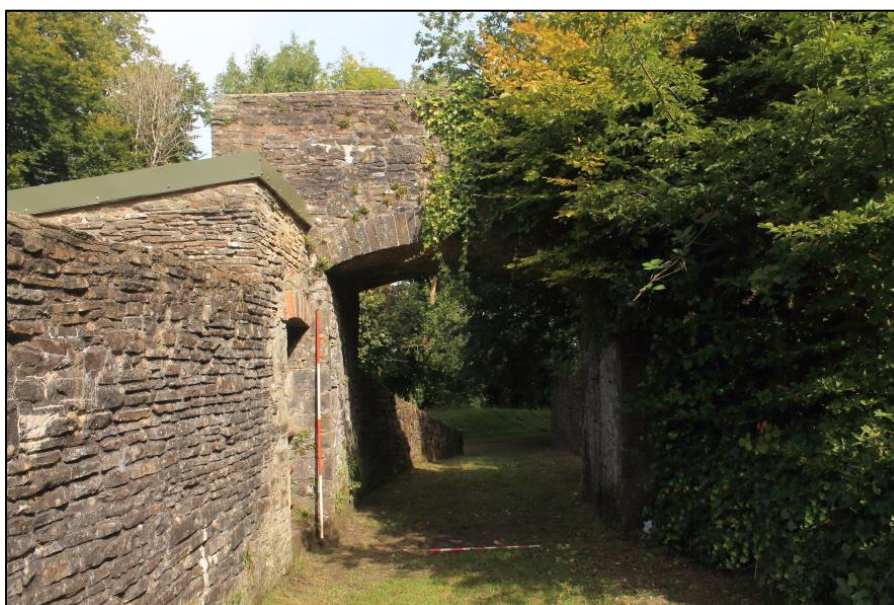
Photo 75: View north of the archway entrance to the rear service yard.
