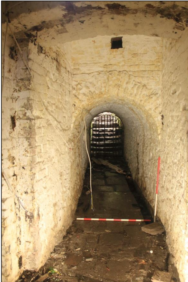
Photo 26: View north looking down the corridor to Entrance 2.
