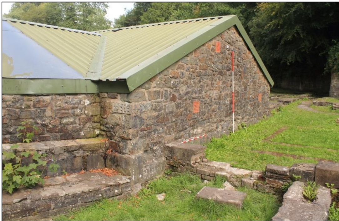
Photo 49: View northeast of the south wall of the former drawing room, showing the lower course of dressed stone. 2m and 1m scales.
