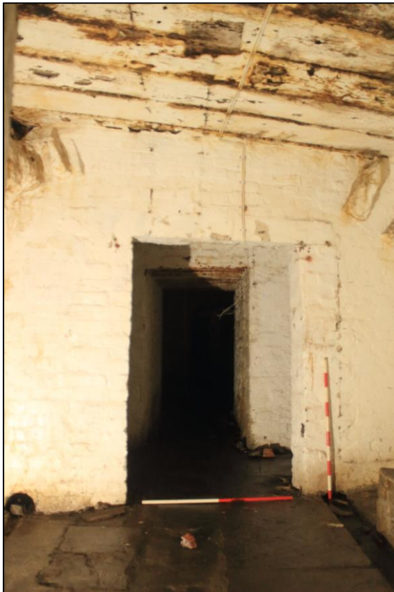
Photo 24: View south from Room 4, looking from Compartment B, through Compartment A and into Corridor 2, showing the timber ceiling and remnants of the masonry arched ceiling in the inserted brick wall.
