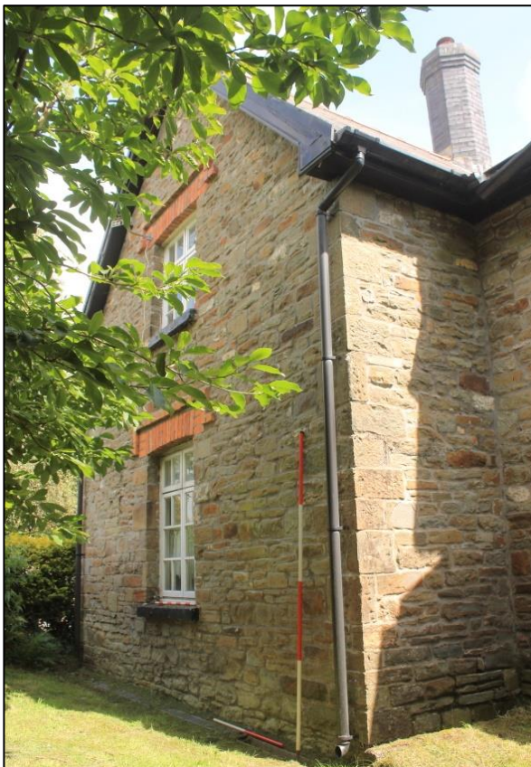
Photo 90: View northeast of the west elevation of Pond Cottage.
