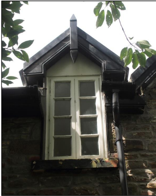
Photo 89: View west of detail of stairway window on east elevation.
