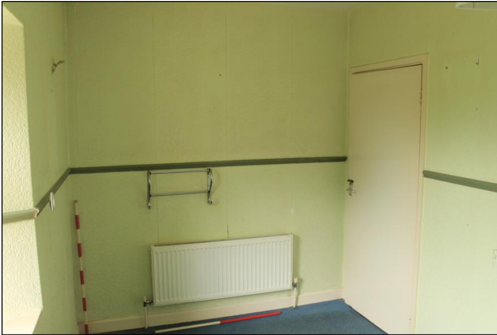
Photo 110: View west of the entry to the first floor bathroom. 1m scales.
