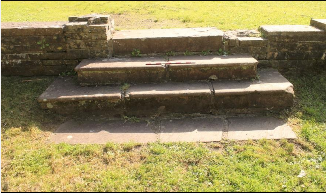
Photo 46: View east of stone steps leading down to the lower terrace. 0.5m scale.
