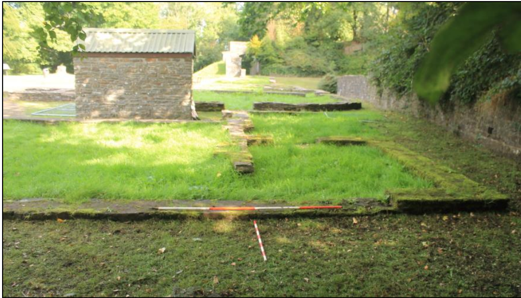
Photo 52: View north over rooms at the east end of Gnoll House, including a former scullery and dairy. 2m and 1m scales.
