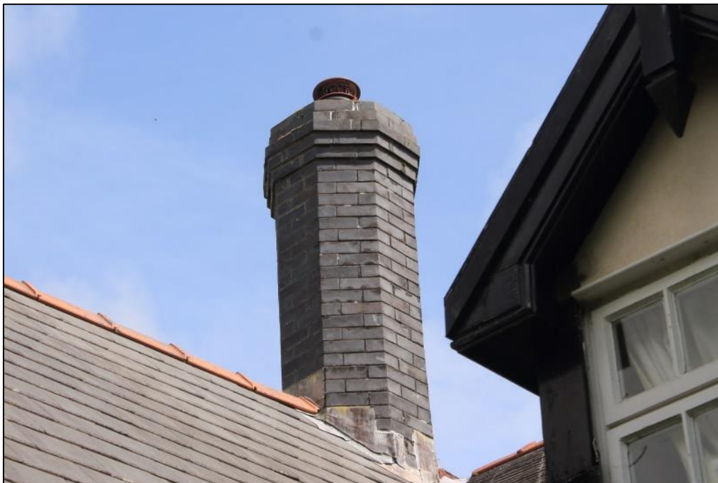
Photo 82: View northeast of the octagonal chimney.
