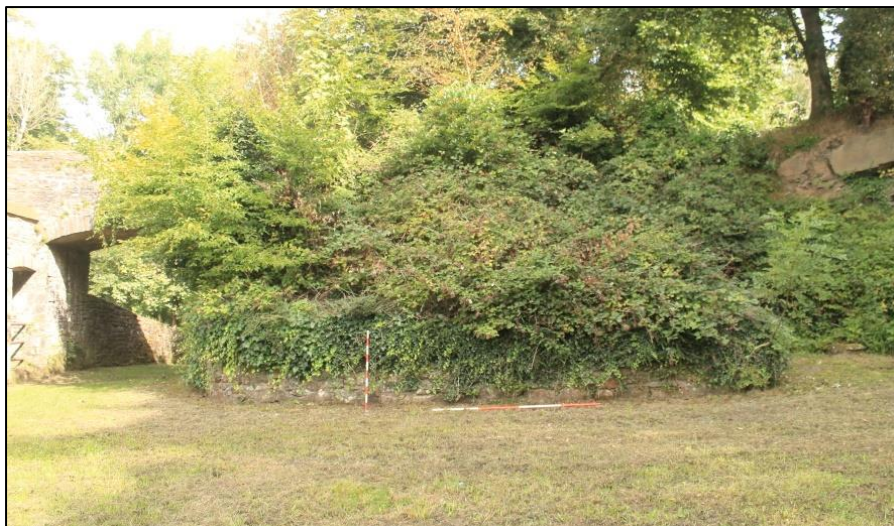
Photo 74: View north showing the retaining wall running up the entrance structure on the left.
