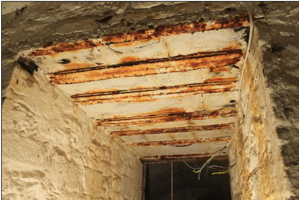
Photo 18: View north of the roof structure in Corridor 2.
