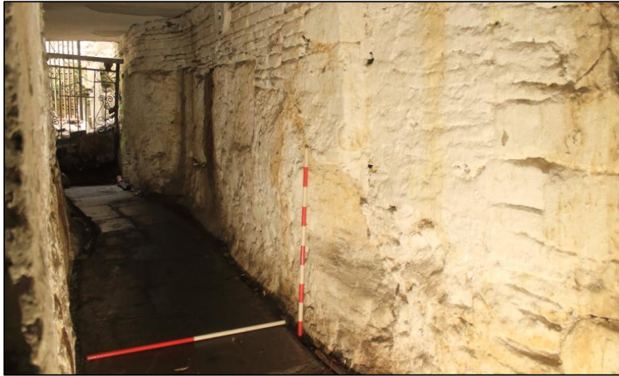
Photo 33: View southeast of the western wall of Corridor 4 showing the vertical butt joint and rock-cut walling. 1m scales.
