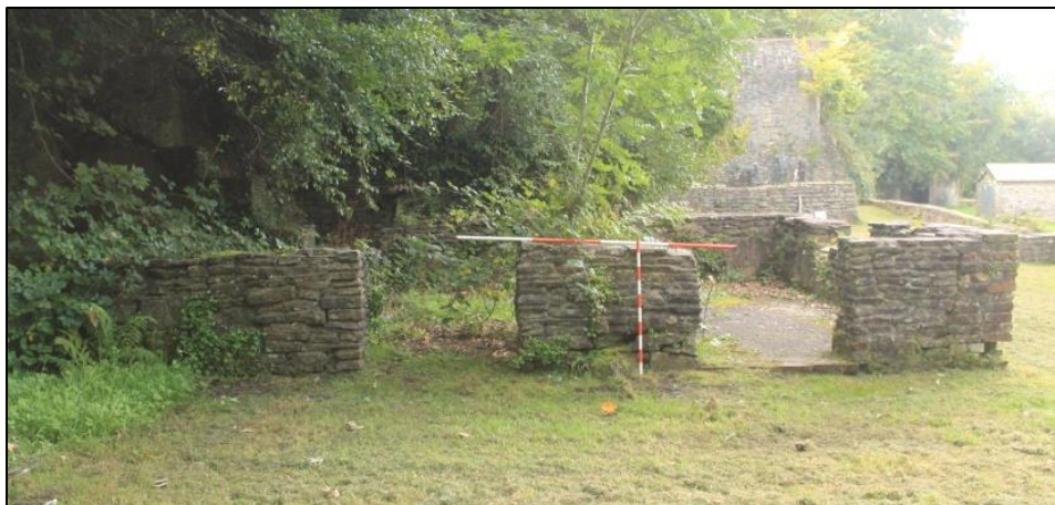
Photo 68: View south of the northern wall of the detached room.
