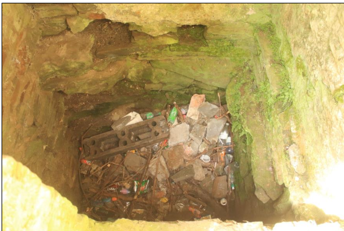
Photo 79: View west of the interior of the former w.c.
