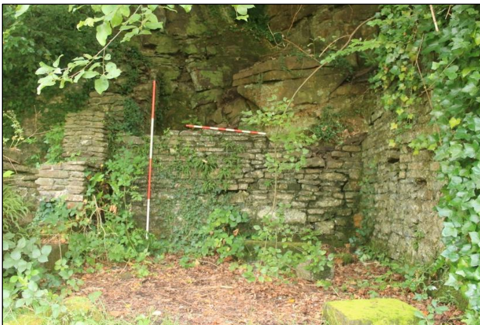
Photo 70: View east of the smaller of the two detached rooms against the rock face to the east of Gnoll House.
