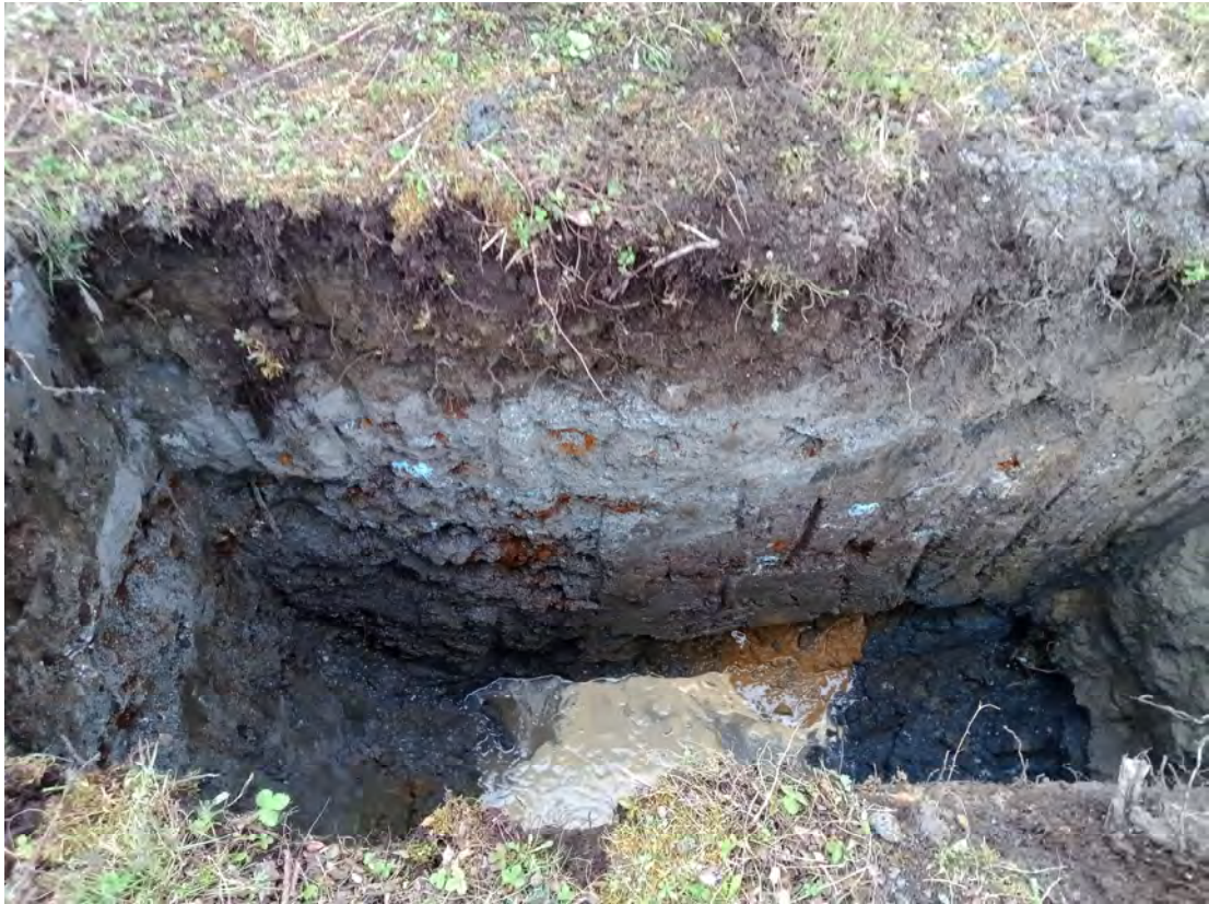
Photograph 5: Excavation at TP12.
