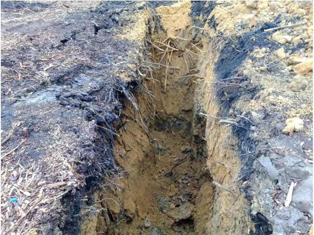
Photograph 1: Excavation at TP03.
