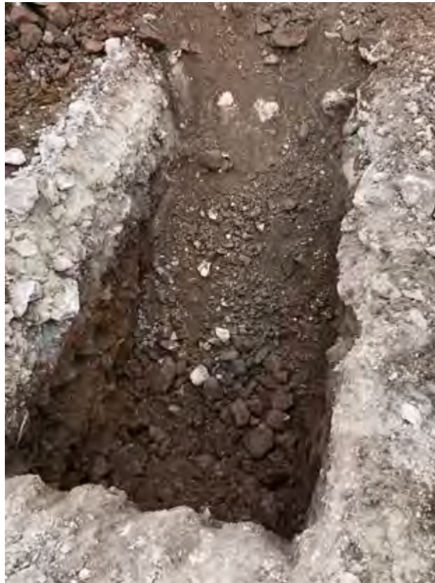
Photograph 25: View of trial pit, TP218.
