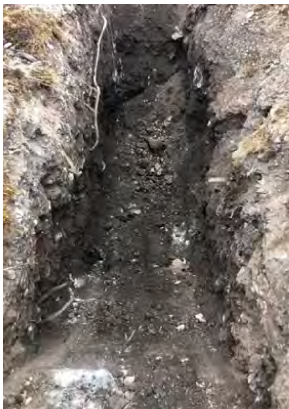
Photograph 9: View of trial pit, TP208A.
