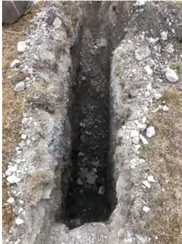
Photograph 3: View of trial pit, TP204.
