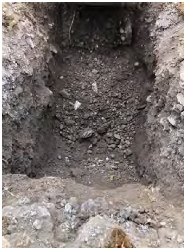
Photograph 23: View of trial pit, TP217.
