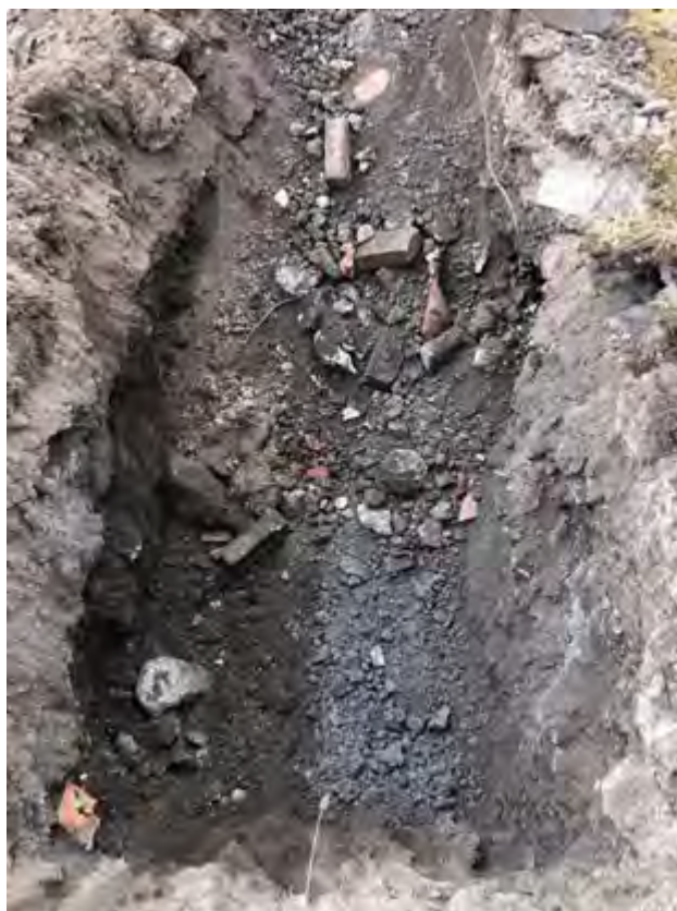
Photograph 19: View of trial pit, TP215.
