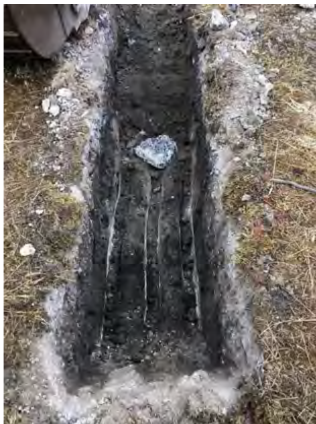
Photograph 7: View of trial pit, TP208.
