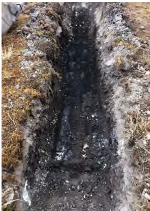
Photograph 15: View of trial pit, TP213.
