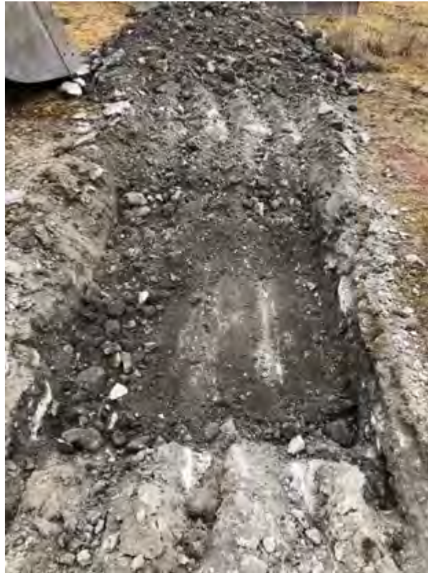
Photograph 21: View of trial pit, TP216.
