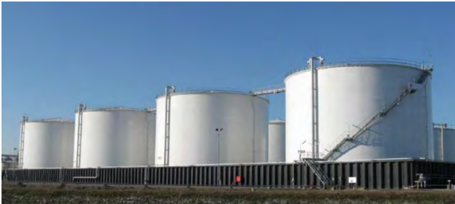
Figure 45 – Typical vessels for the storage of feedstock ethanol in a bunded compound.
