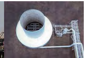
Figures 52 to 55 – Details of ground flares used in other similar facilities.
