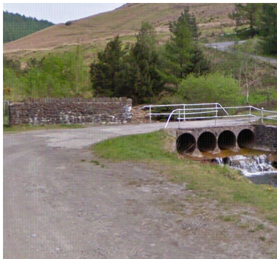
Existing Pipe Bridge Crossing Photo
