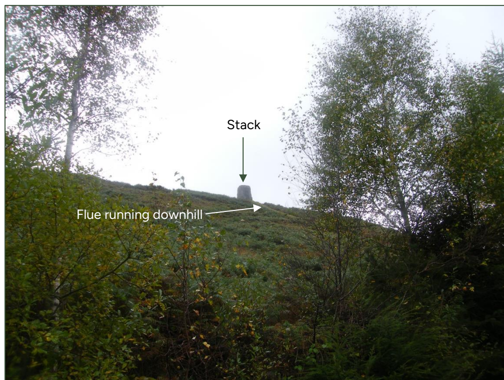
Photo 1: Cwm Pelenna Colliery Ventilation Furnace and Stack from Fforch-Dwm Road
