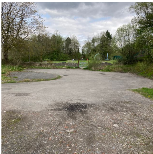
Figure 9. Tarmac area at the northern end of the Site.
