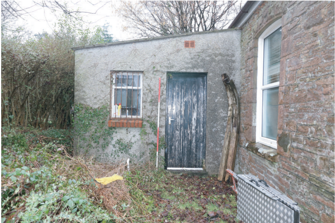
Plate 85. Ebenezer Chapel, Rhos - Earlier Chapel. Kitchen extension attached to NE corner of Sunday School building. West facing elevation. Looking E.
