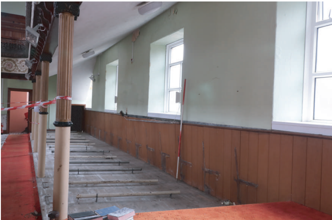
Plate 36. Ebenezer Chapel, Rhos - Interior view of north aisle. Looking W.
