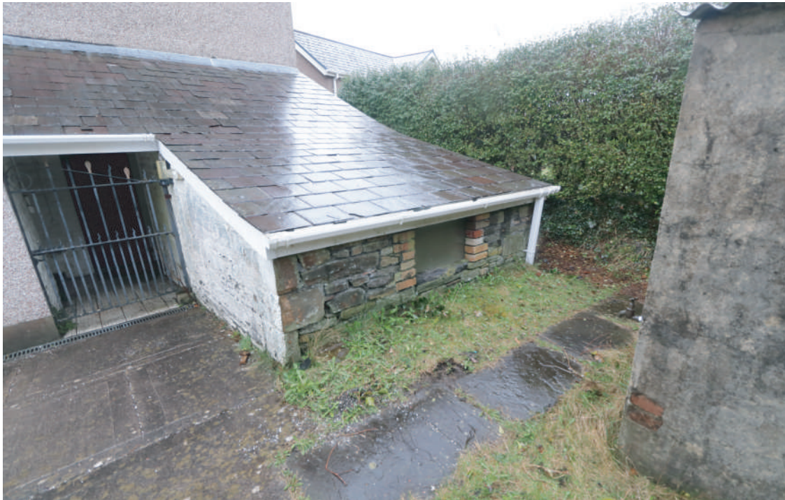
Plate 20. Ebenezer Chapel, Rhos - Rear extension at NE corner of rear of chapel (Store Room). Looking NW.
