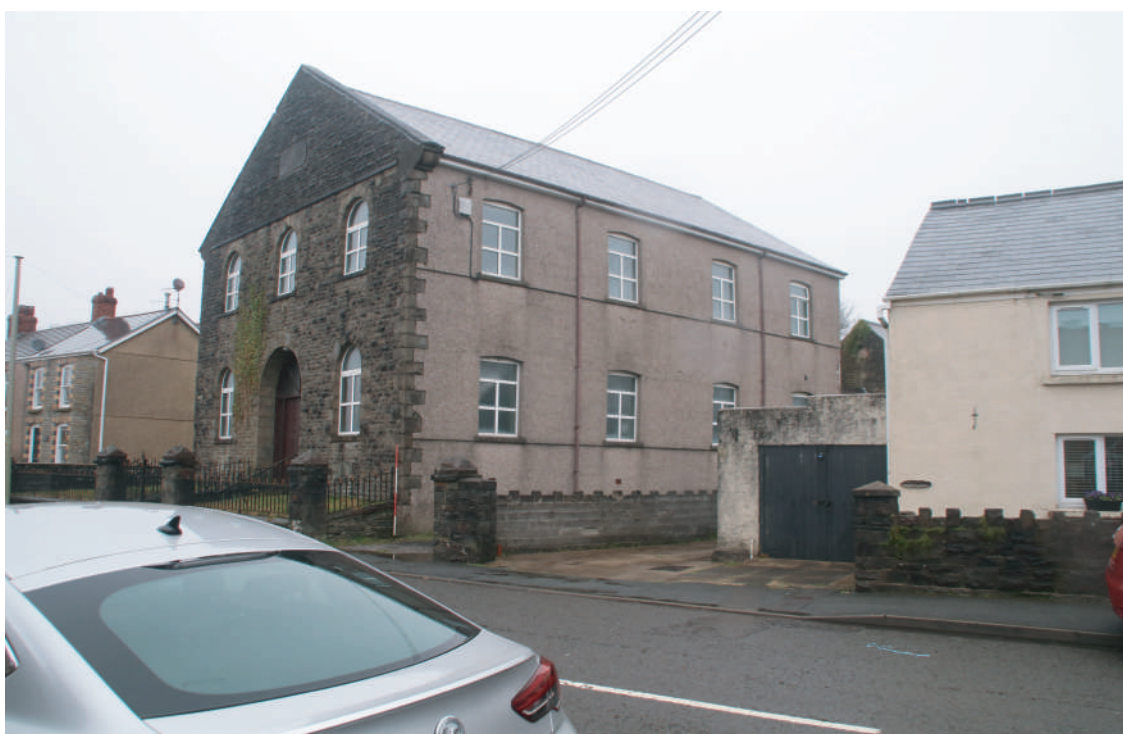
Plate 03. Ebenezer Chapel, Rhos - Ebenezer Chapel front west facing and south facing elevation from Neath Road. Looking NE.
