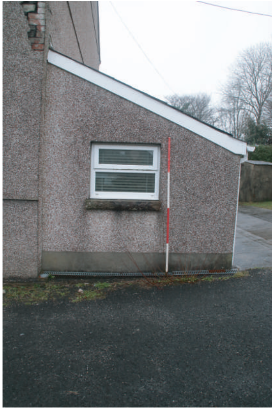
Plate 18. Ebenezer Chapel, Rhos - Side view of rear kitchen extension. Looking N.
