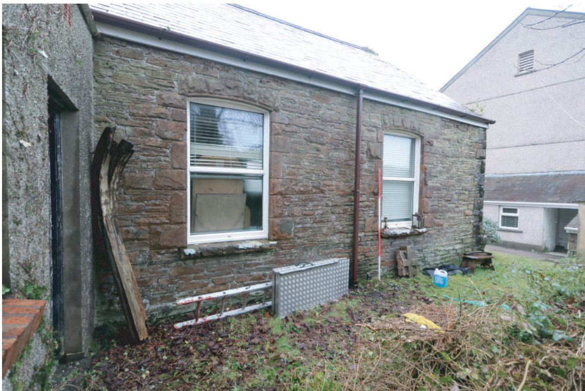
Plate 86. Ebenezer Chapel, Rhos - Earlier Chapel. North facing elevation. Looking SW.
