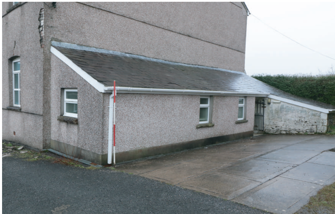
Plate 18. Ebenezer Chapel, Rhos - Rear kitchen extension against east facing rear elevation. Looking NW.
