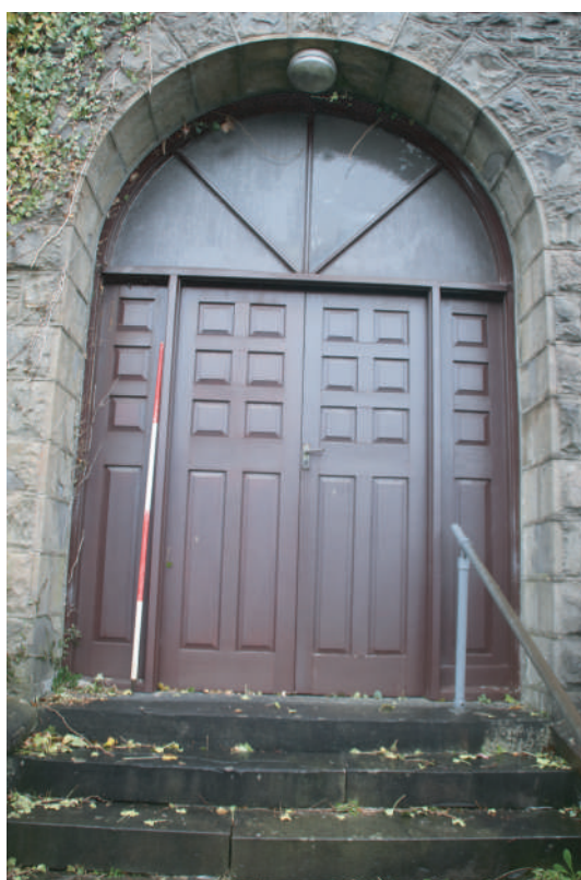
Plate 27. Ebenezer Chapel, Rhos - Front entrance into Chapel. Looking E.
