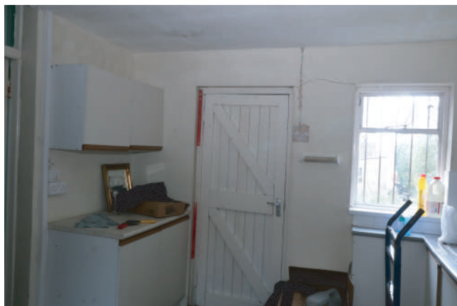
Plate 94. Ebenezer Chapel, Rhos - Earlier Chapel. Kitchen. Looking W.
