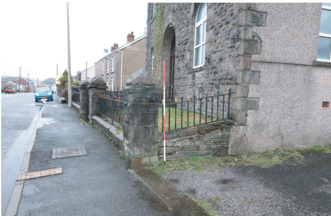
Plate 08. Ebenezer Chapel, Rhos - Stone walling and wrought iron railings at front of chapel. Looking N.
