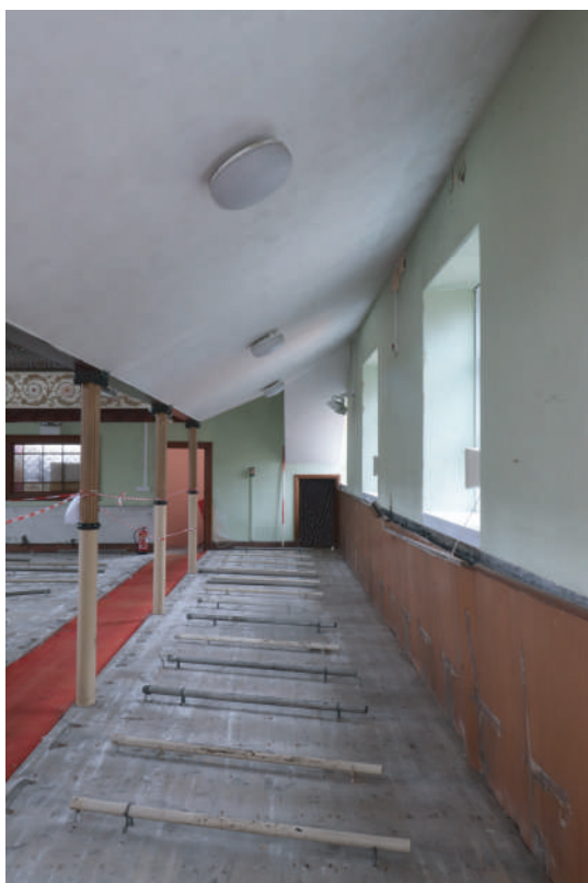
Plate 32. Ebenezer Chapel, Rhos - Interior view of north aisle. Looking W.
