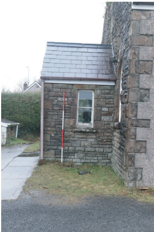
Plate 82. Ebenezer Chapel, Rhos - Earlier Chapel. South facing elevation of porch. Looking N.
