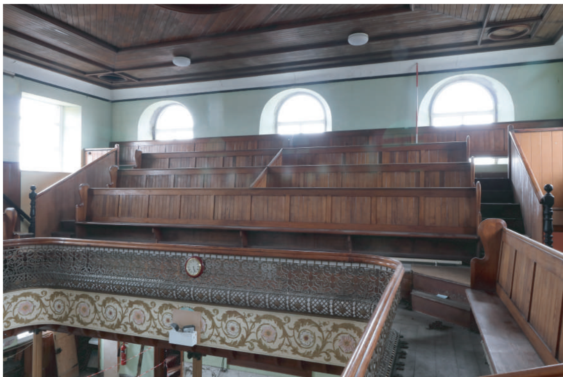
Plate 61. Ebenezer Chapel, Rhos - Interior view from Balcony area. Looking W.
