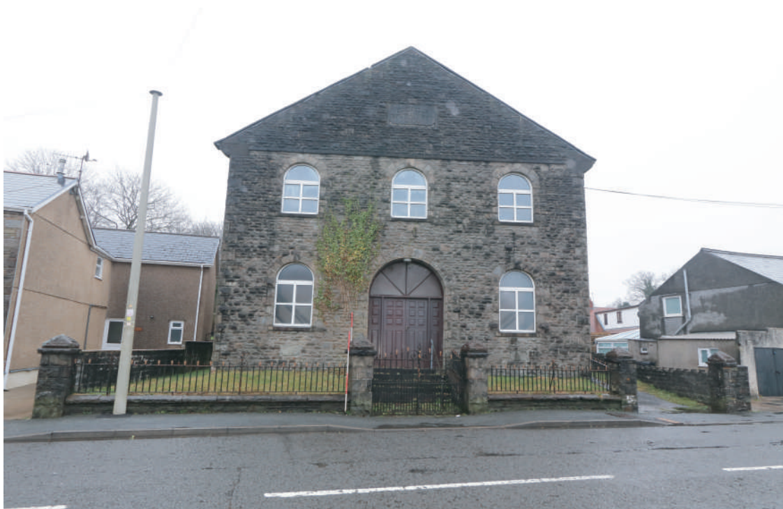
Plate 06. Ebenezer Chapel, Rhos - Ebenezer Chapel front west facing elevation from Neath Road. Looking E.
