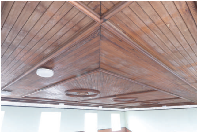
Plate 67. Ebenezer Chapel, Rhos - Interior view of decorative timber ceiling. Looking NE.
