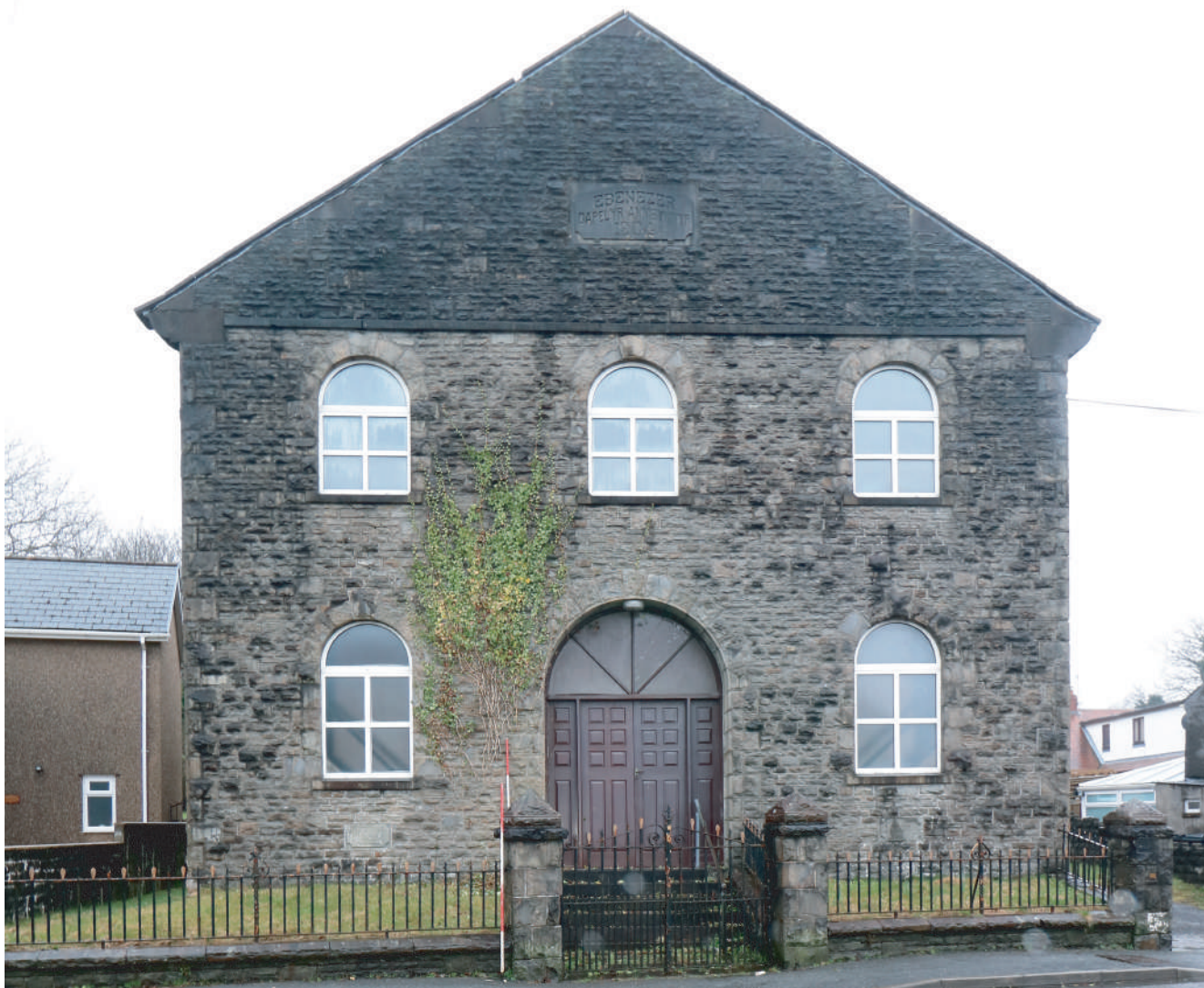
Plate 07. Ebenezer Chapel, Rhos - Ebenezer Chapel front west facing elevation from Neath Road. Looking E.
