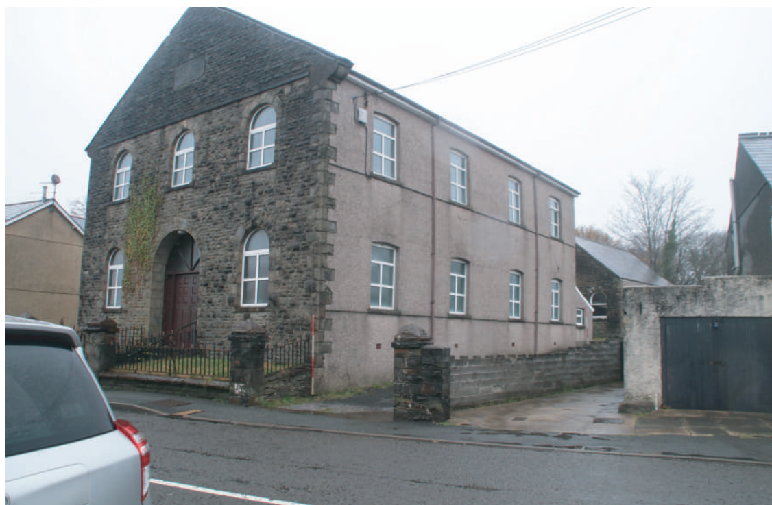
Plate 04. Ebenezer Chapel, Rhos - Ebenezer Chapel front west facing and south facing elevation from Neath Road. Looking NE.
