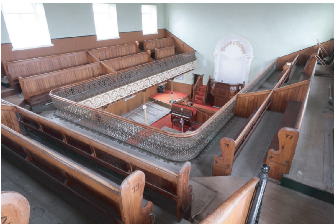
Plate 55. Ebenezer Chapel, Rhos - Interior view from Balcony area. Looking NE.
