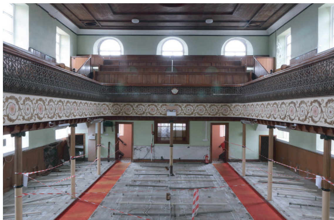
Plate 40. Ebenezer Chapel, Rhos - Interior view of Nave from podium/sanctuary. Looking W.
