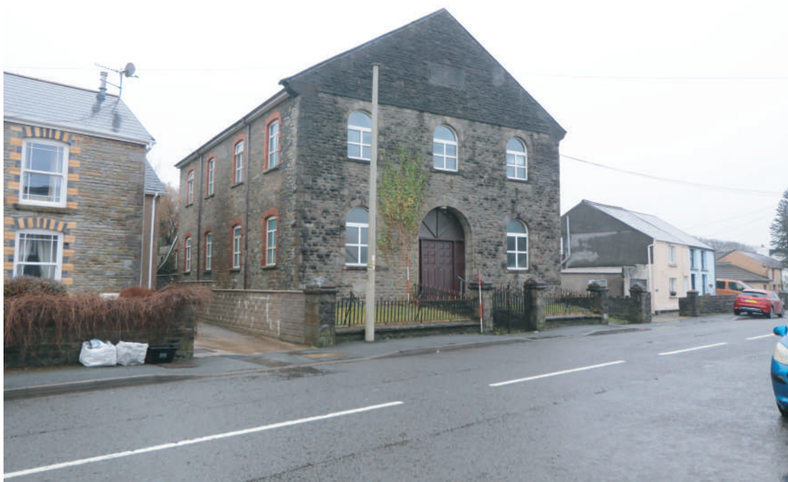
Plate 05. Ebenezer Chapel, Rhos - Ebenezer Chapel front west facing and north facing elevation from Neath Road. Looking SE.
