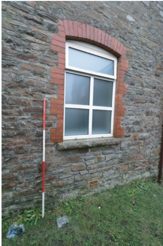
Plate 21 Ebenezer Chapel, Rhos - Side north facing elevation window detail. Looking SW.
