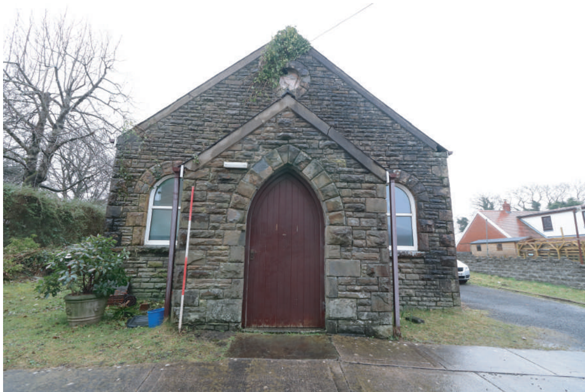
Plate 79. Ebenezer Chapel, Rhos - Earlier Chapel used as Sunday School. Front west facing elevation. Looking E.
