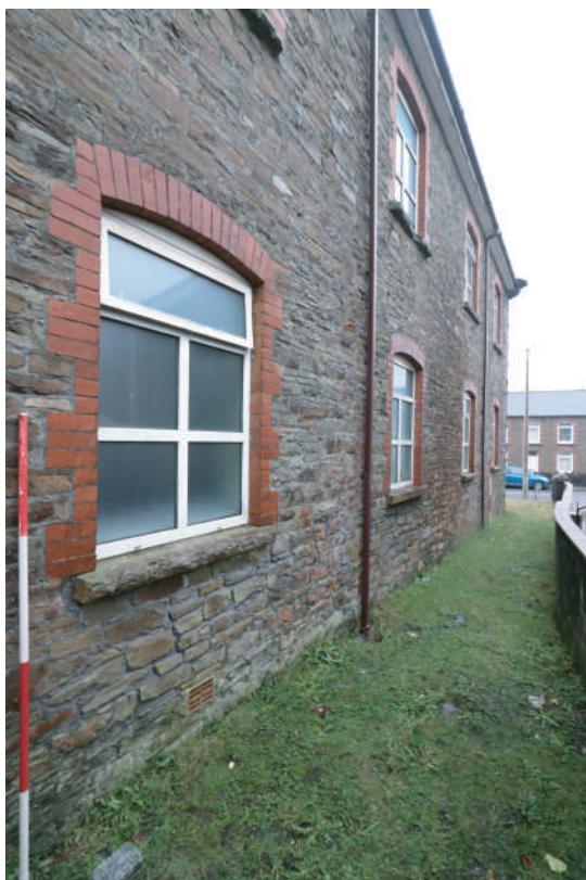
Plate 24 Ebenezer Chapel, Rhos - Side north facing elevation window detail. Looking W.
