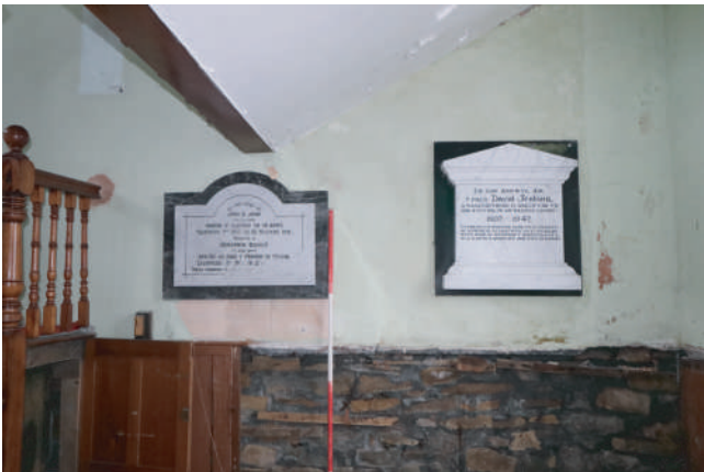
Plate 46. Ebenezer Chapel, Rhos - Memorial plaques to David Jenkins, John John and Benjamin Davies against the east wall in southern aisle. Looking E.
