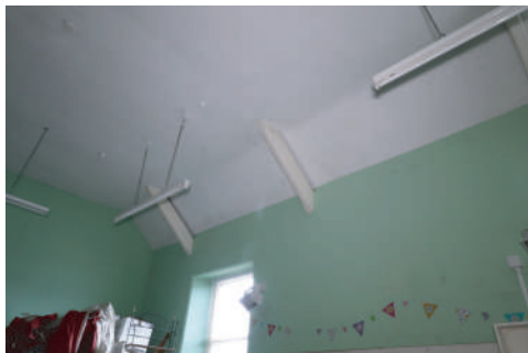
Plate 92. Ebenezer Chapel, Rhos - Detail of ceiling within Sunday School building. Looking NW.
