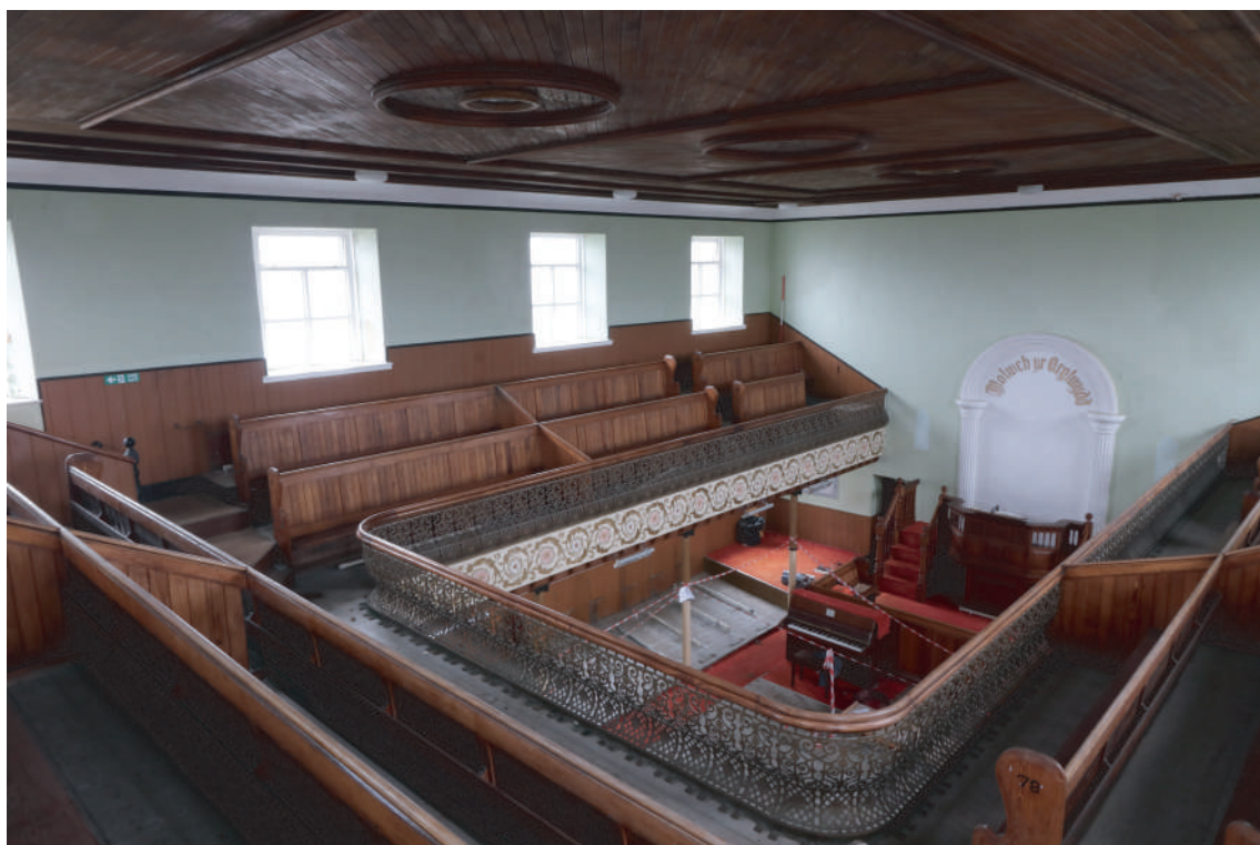
Plate 59. Ebenezer Chapel, Rhos - Interior view from Balcony area. Looking NE.
