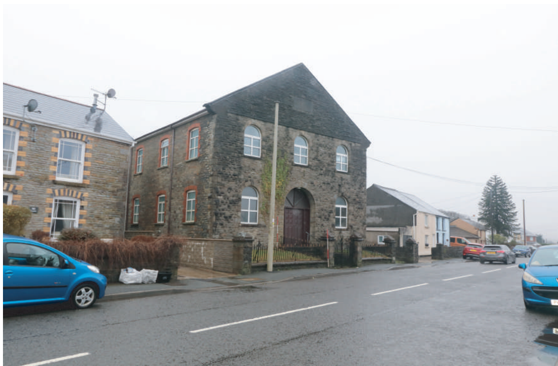
Plate 02. Ebenezer Chapel, Rhos - Ebenezer Chapel front west facing and north facing elevation from Neath Road. Looking SE.
