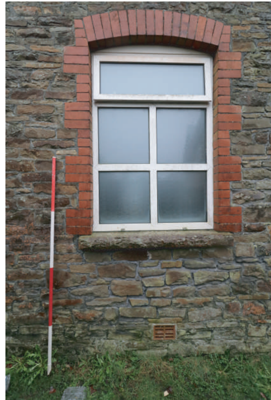
Plate 22. Ebenezer Chapel, Rhos - Side north facing elevation window detail. Looking W.
