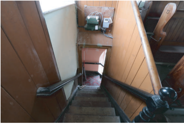
Plate 65. Ebenezer Chapel, Rhos - Interior view of access stairs from balcony to entrance hall on S side of hall. Looking west.
