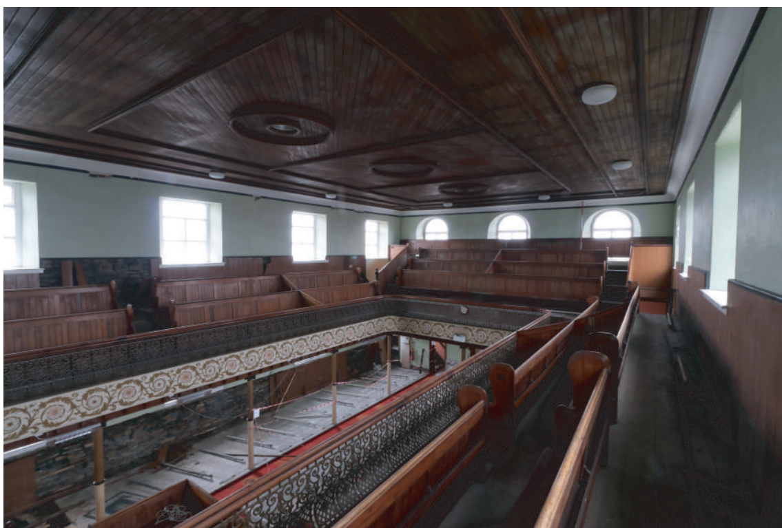
Plate 60. Ebenezer Chapel, Rhos - Interior view from Balcony area. Looking SW.
