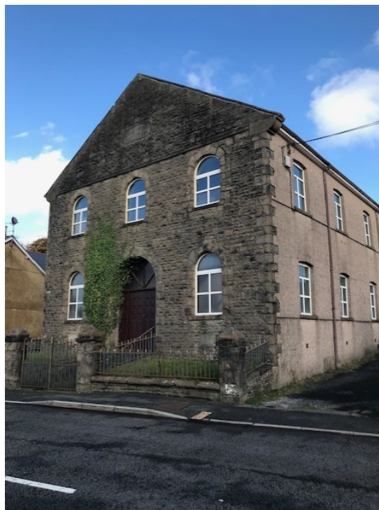
Photograph shows front Elevation of Former Chapel, fronting Neath Road
