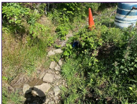
Discharge pipe (W19) into watercourse/drainage ditch W2
