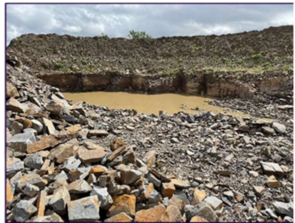
Current south-eastern corner secondary sump
