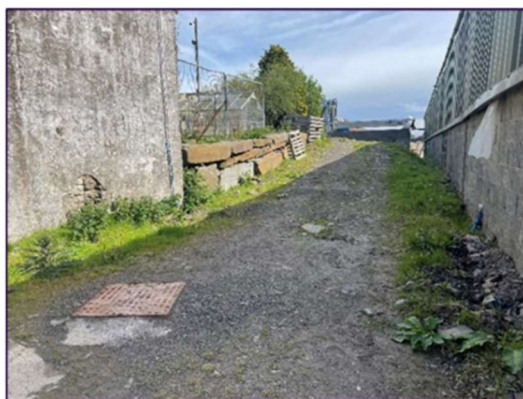
Route of culverted pipeline (W6) through processing area with access manhole
