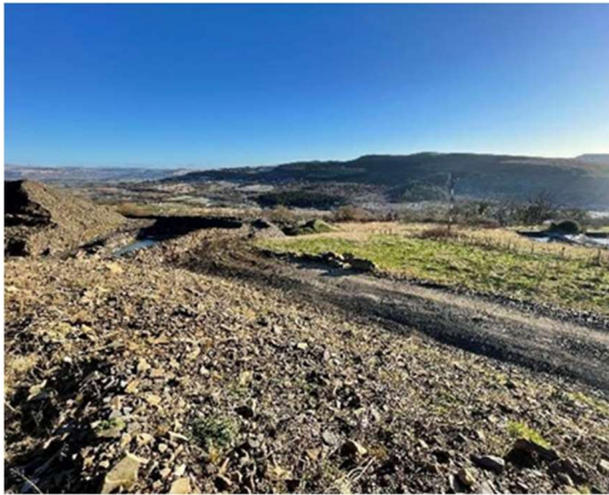
View of southern restored area looking east, from haul road.
