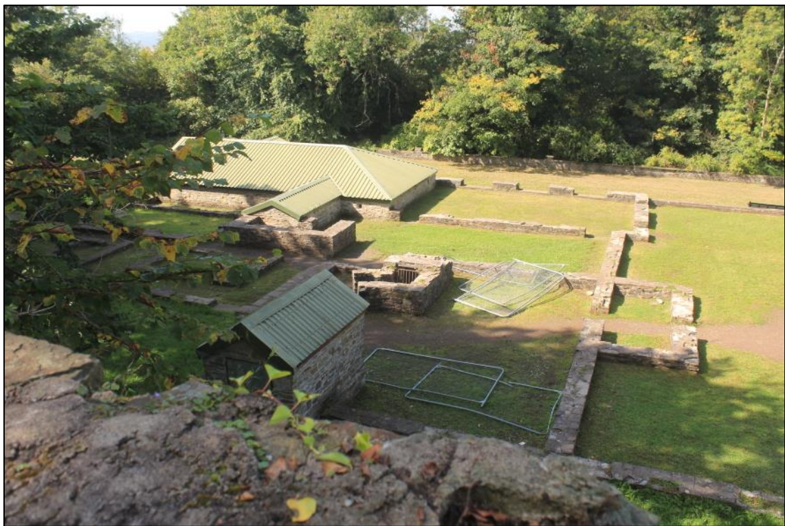
Photo 1: View west over the Gnoll House ruins. The roofed buildings cover cellars and their entrances.
