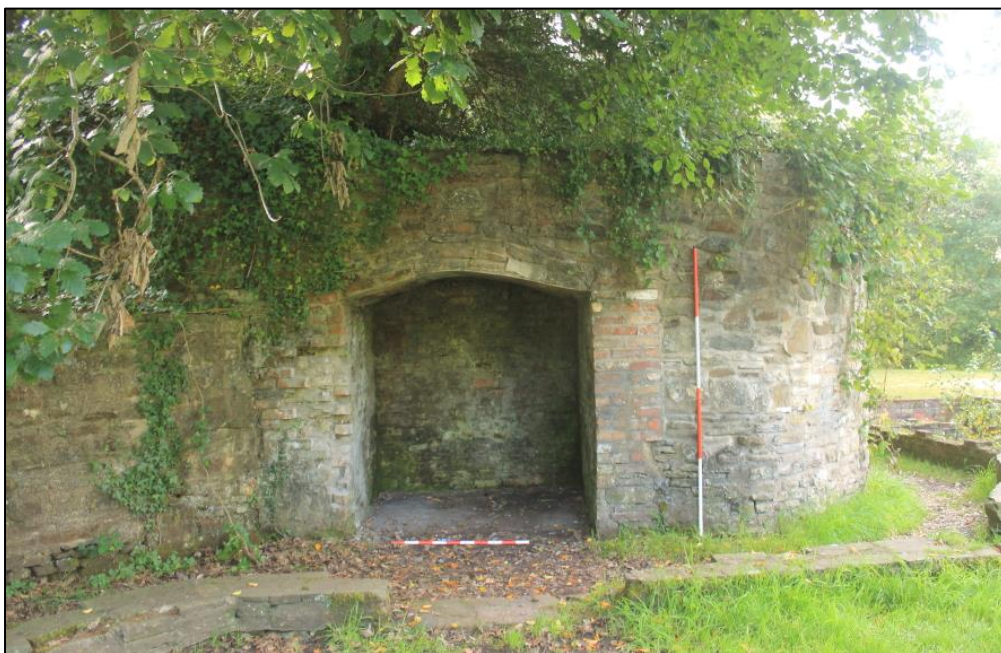
Photo 61: View south of a small room within the retaining wall adjacent to the house. 2m and 1m scales.
