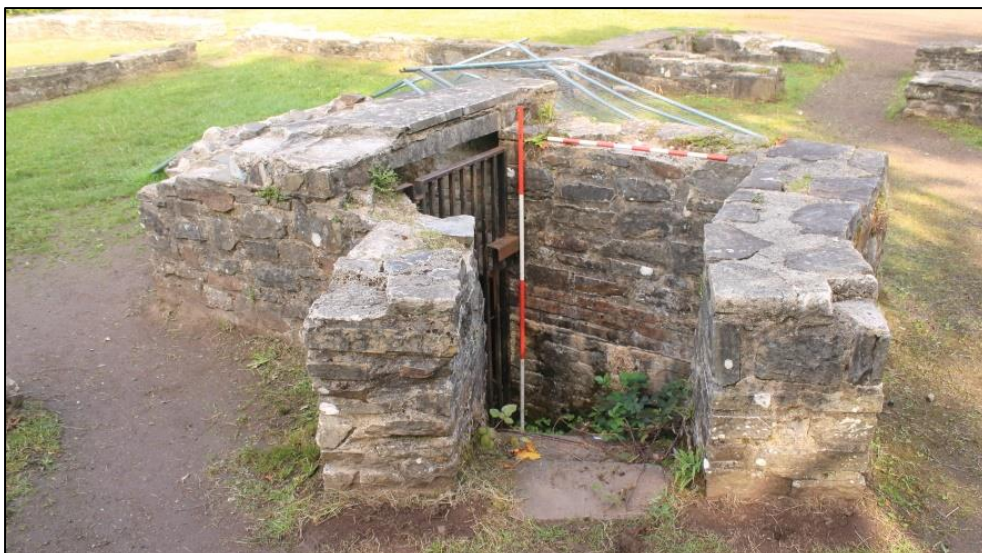
Photo 34: View northwest of Entrance 3 at surface level. 2m scale.
