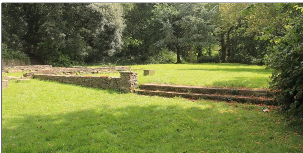
Photo 55: View southeast showing the retaining wall and steps to the west of the former conservatory. 2m and 1m scale.
