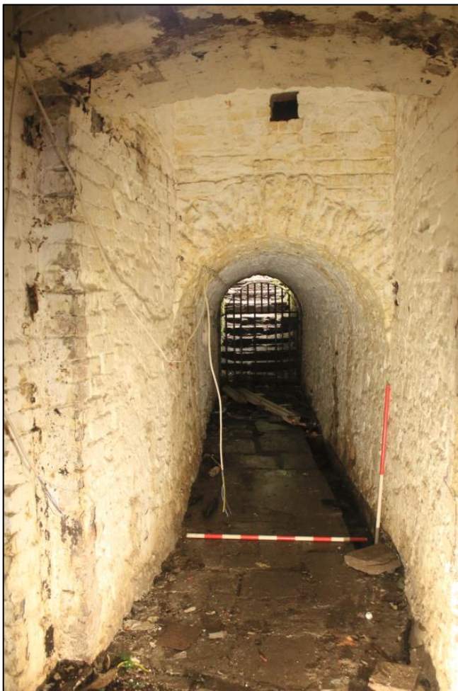
Photo 26: View north looking down the corridor to Entrance 2. 1m scales.
