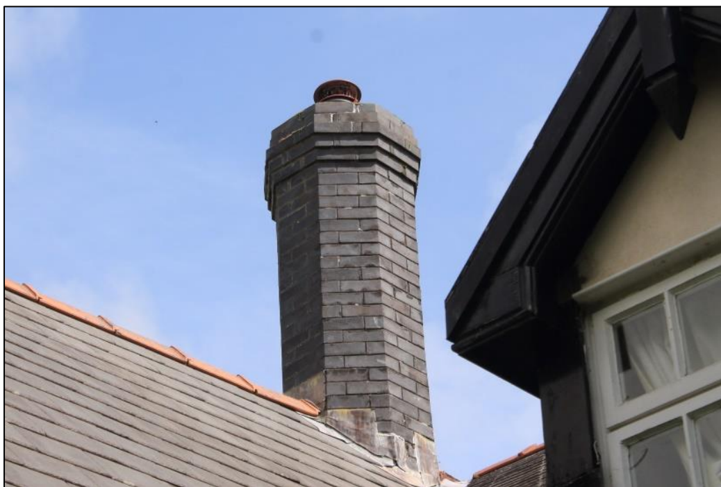
Photo 82: View northeast of the octagonal chimney.
