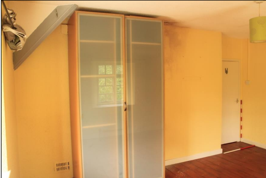
Photo 112: View east of Bedroom 1 with the vent in a possible former fireplace to the lower left. 1m scales.
