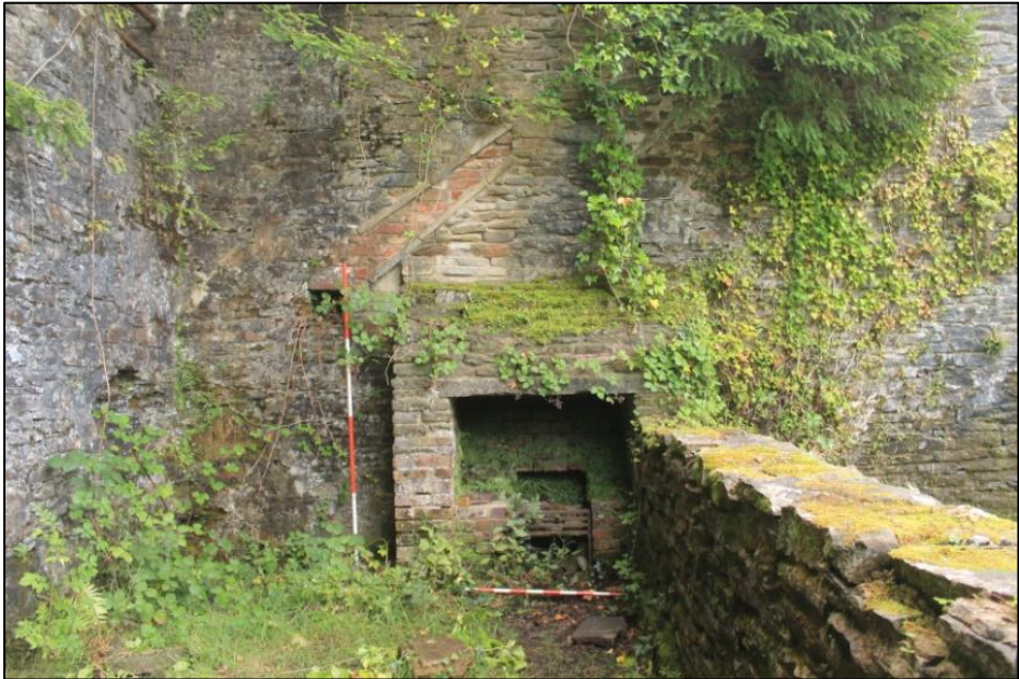
Photo 64: View south of the fireplace within the former washhouse. 2m and 1m scales.
