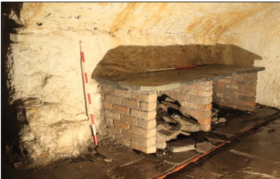
Photo 38: View northwest of shelving within Room 5. 1m scales.
