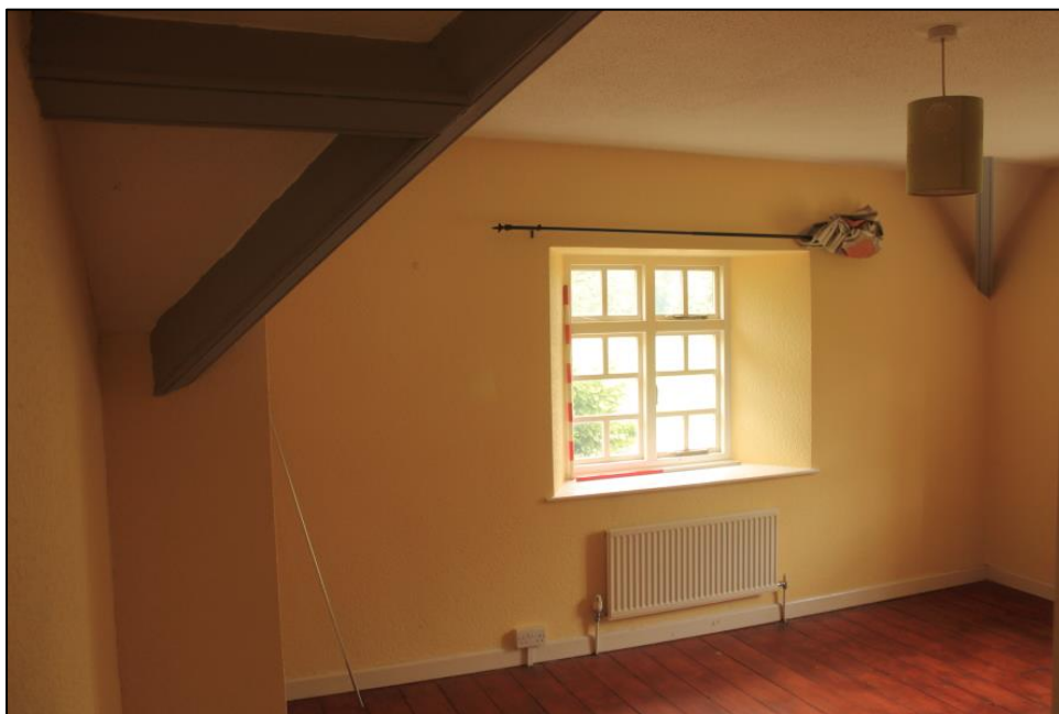
Photo 111: View west in Bedroom 1. 1m scales.
