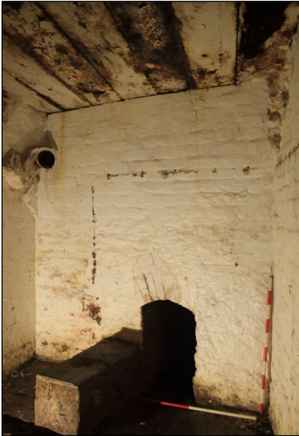
Photo 22: View west of the opening in the west wall of Room 4 (Compartment B).
