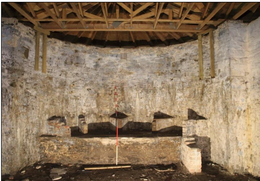
Photo 6: View west of bay front of Room 1. 1m scales.
