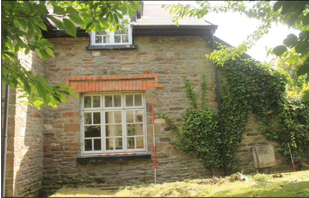
Photo 91: View east of the rear west elevation of Pond Cottage. 2m scale.
