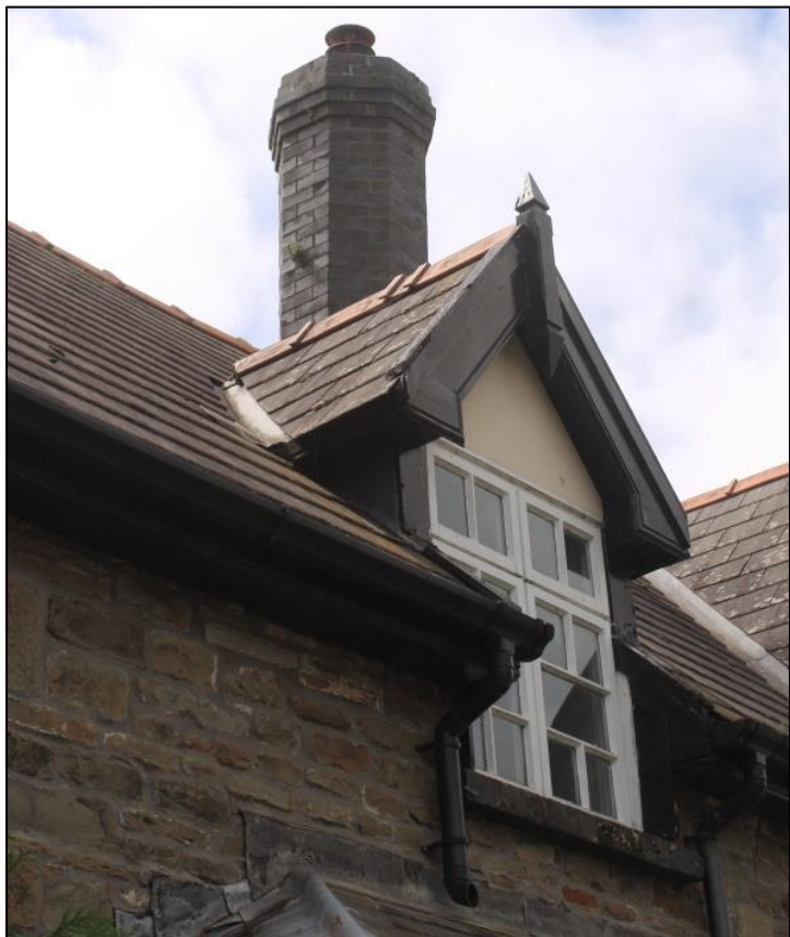
Photo 86: View southwest. First floor dormer window and roofing detail.
