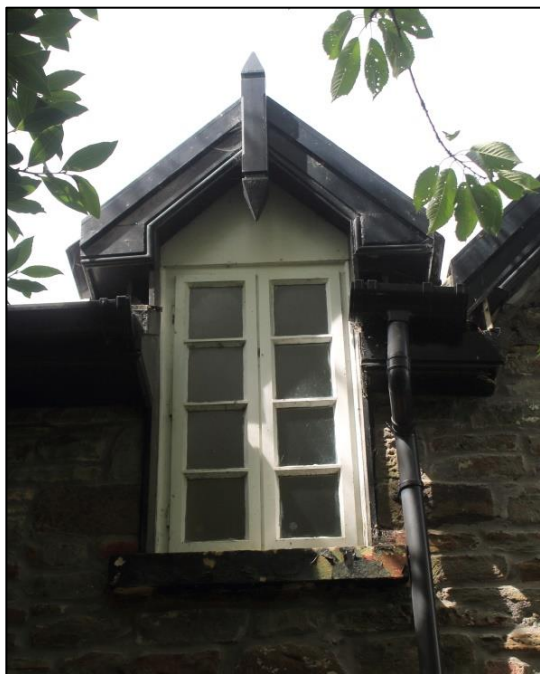
Photo 89: View west of detail of stairway window on east elevation.
