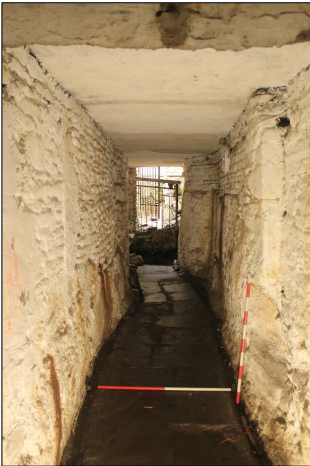
Photo 32: View south, looking down Corridor 4 towards Entrance 3. 1m scales.
