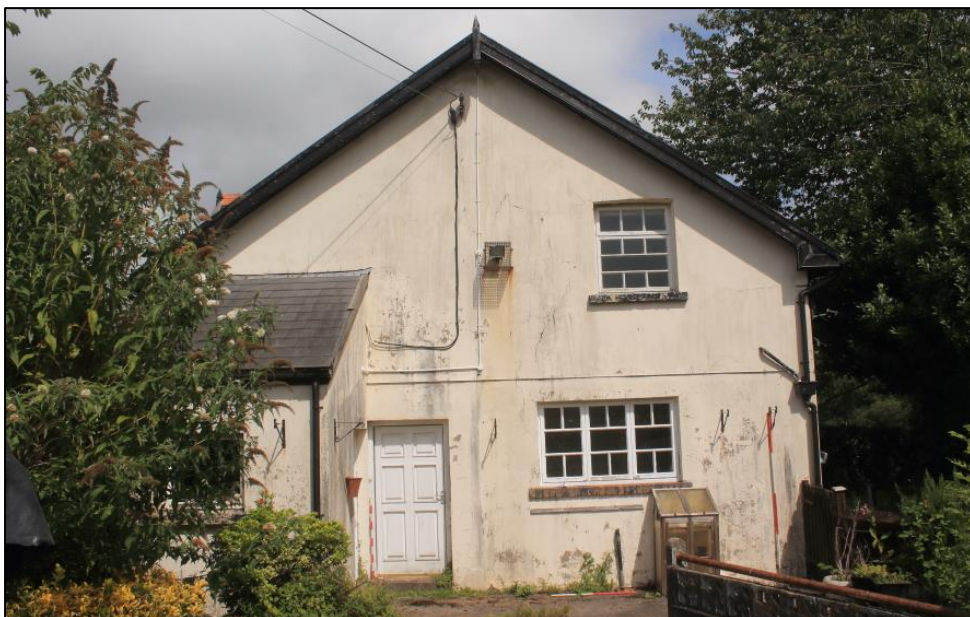
Photo 92: View north of the rear, south elevation of Pond Cottage. 2m and 1m scales.
