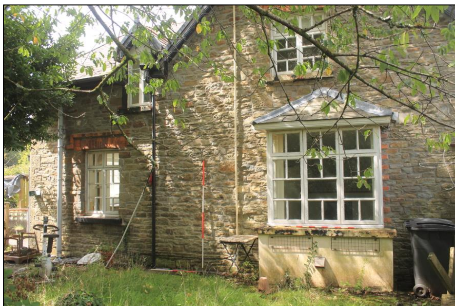
Photo 87: View west of the east elevation of Pond Cottage. 2m and 1m scales.
