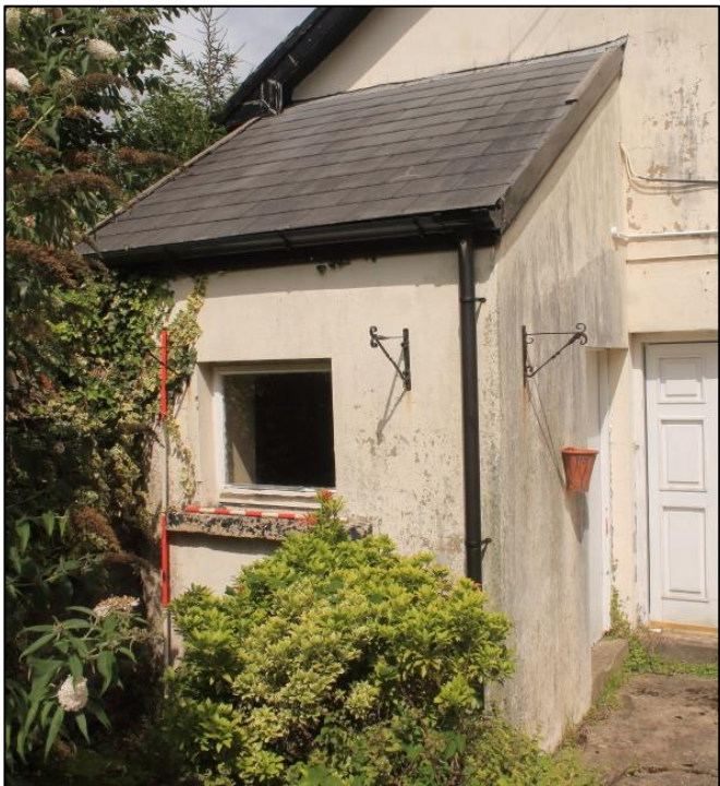
Photo 93: View northwest of the rear lean-to attachment. 2m and 1m scales.
