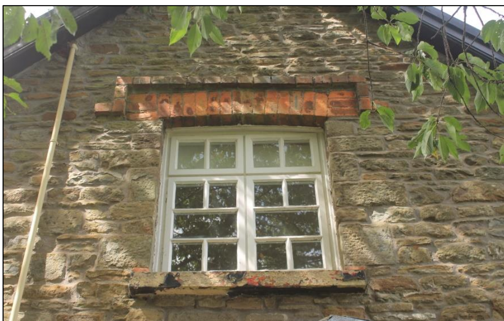
Photo 88: View west showing the detail of first floor window on east elevation.
