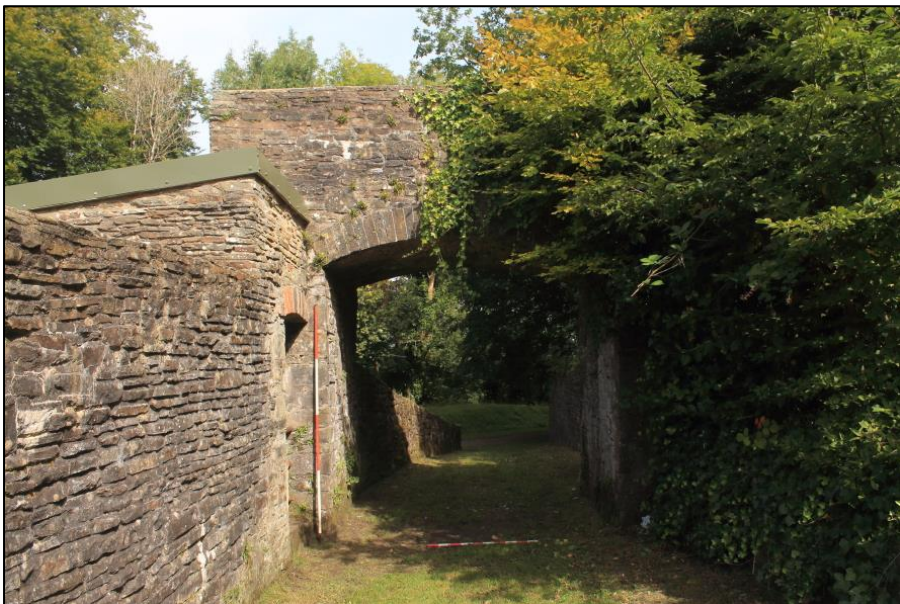
Photo 75: View north of the archway entrance to the rear service yard. 2m and 1m scales.
