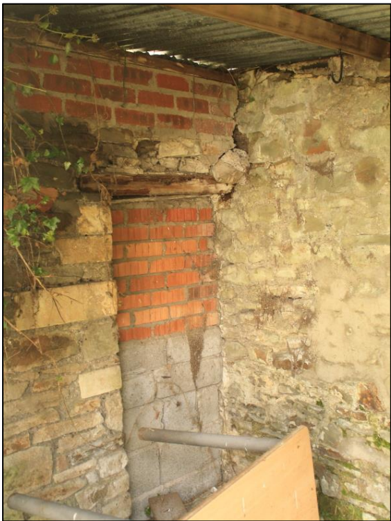
Photo 98: View southeast of blocked doorway through the external boundary wall, within the garden shed.
