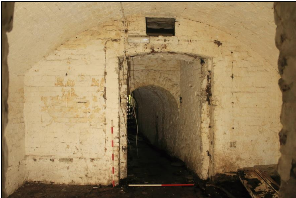
Photo 25: View north from Room 4 (Compartment C) looking into Entrance 2. 1m scales.
