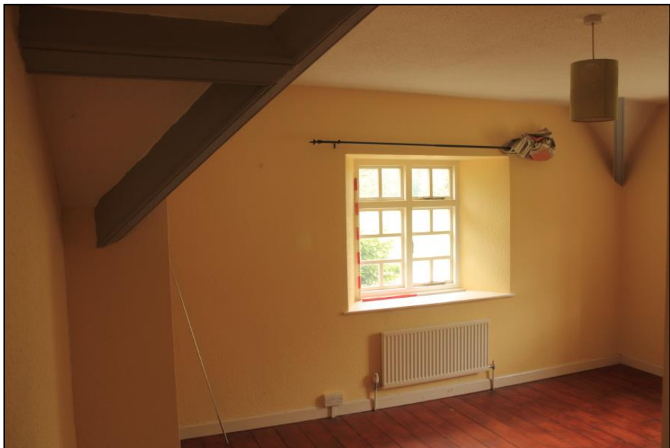
Photo 111: View west in Bedroom 1. 1m scales.
