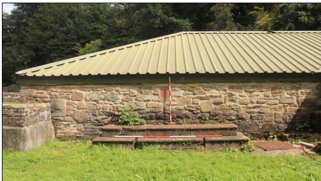
Photo 47: View east of dressed stone steps marking the site of a former window in the library. 2m and 1m scales.
