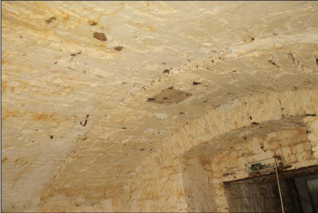
Photo 17: View northwest of changing roof structures at the northern end of Room 3 and entrance to Corridor 2.
