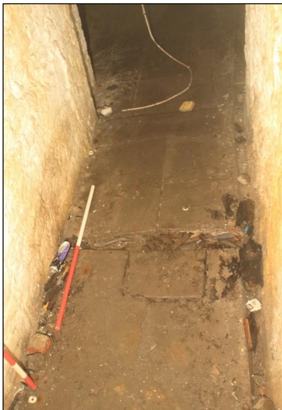
Photo 19: View north of the stone slab floor through Corridor 2.
