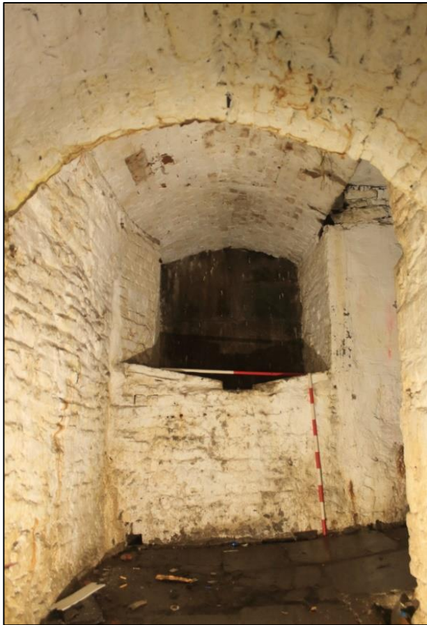
Photo 31: View east of the blocked opening at the eastern end of Corridor 3. 1m scales.
