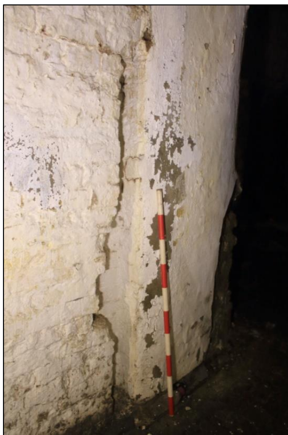
Photo 14: View southeast. Detail of former door jamb between Corridor 1 and Room 2. 1m scale.
