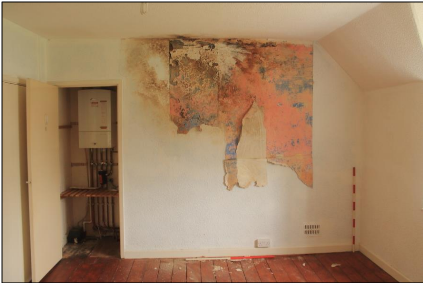
Photo 115: View west in Bedroom 2 showing the airing cupboard to the left and lower vent to the right possible marking a blocked fireplace. 1m scales.
