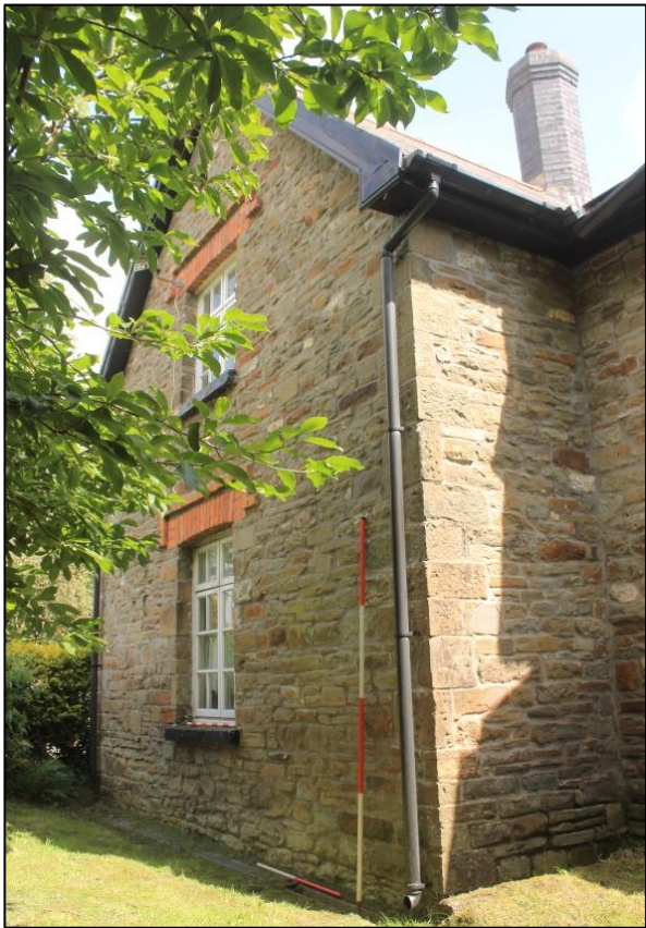
Photo 90: View northeast of the west elevation of Pond Cottage. 2m and 1m scales.
