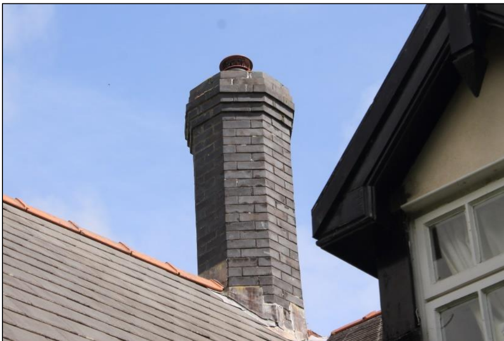
Photo 82: View northeast of the octagonal chimney.
