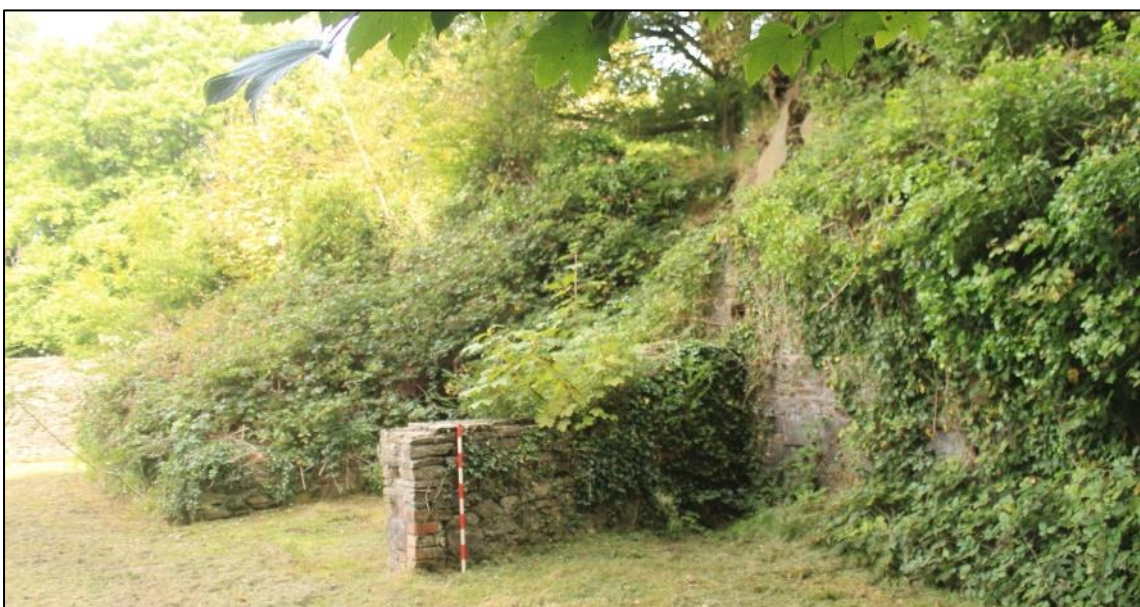
Photo 72: View northwest of walls against the northern side of the service yard area. 1m scale.
