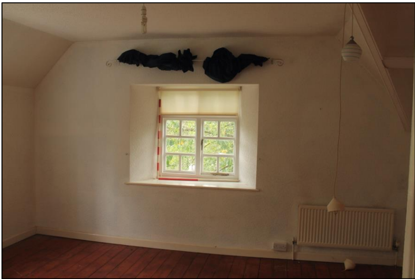
Photo 114: View east in Bedroom 2. 1m scales
