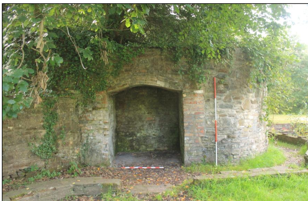
Photo 61: View south of a small room within the retaining wall adjacent to the house. 2m and 1m scales.
