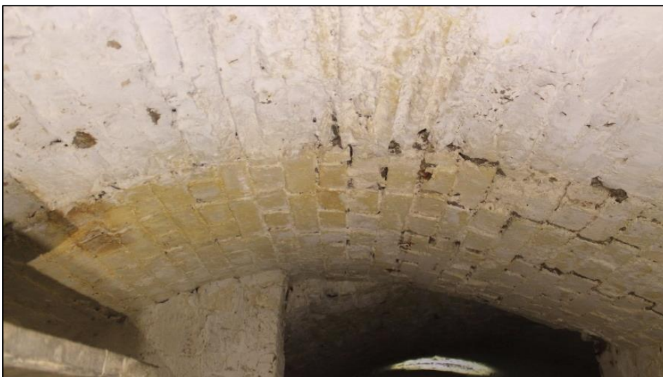
Photo 12: View north, replaced section of roofing in Corridor 1 as it enters Room 3.
