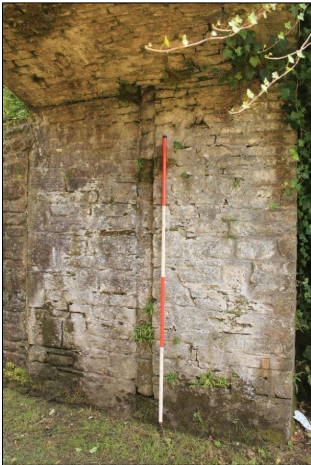
Photo 77: View east of the door jamb groove in the entranceway structure to the service yard. 2m scale.
