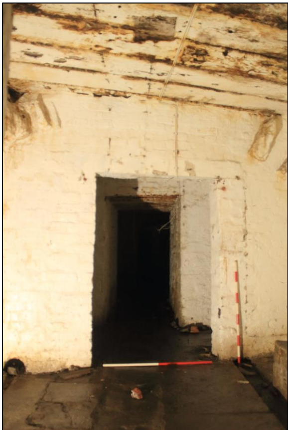
Photo 24: View south from Room 4, looking from Compartment B, through Compartment A and into Corridor 2, showing the timber ceiling and remnants of the masonry arched ceiling in the inserted brick wall. 1m scales.
