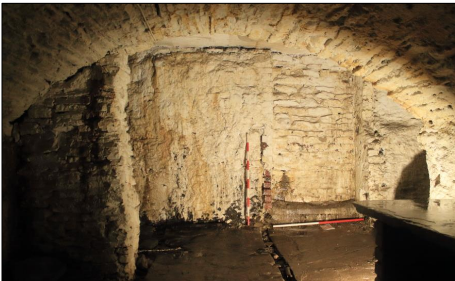
Photo 39: View south out of Room 5 and across Corridor 5, with the blocked doorway visible on the right. 1m scales.
