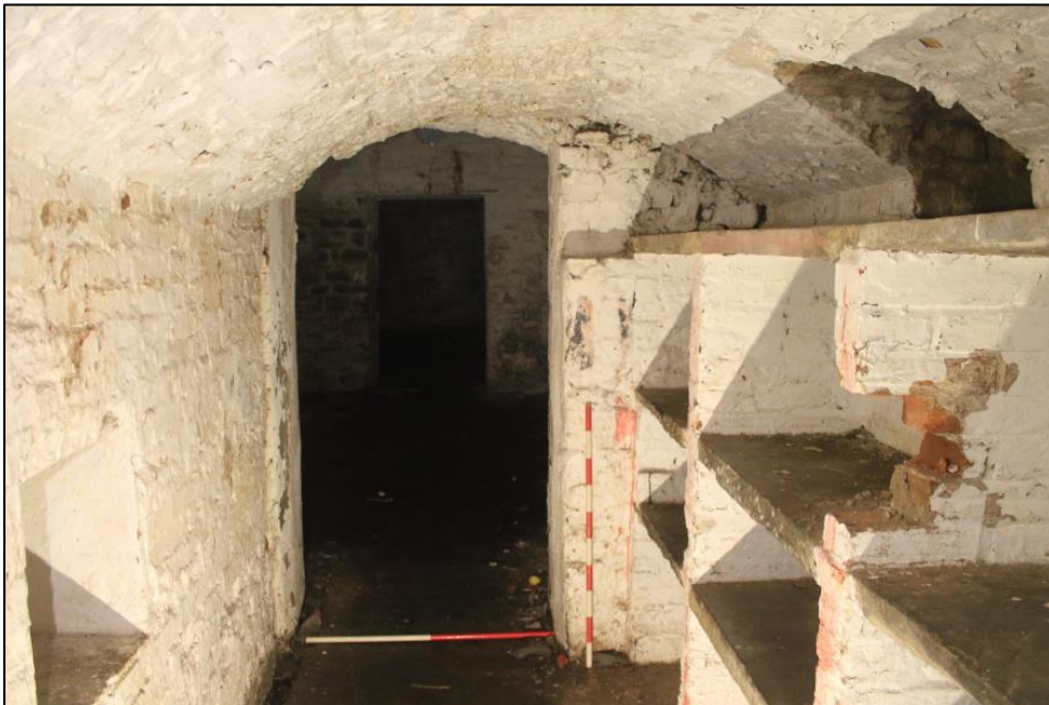
Photo 11: View south down Corridor 1, looking into Room 2. 1m scales.
