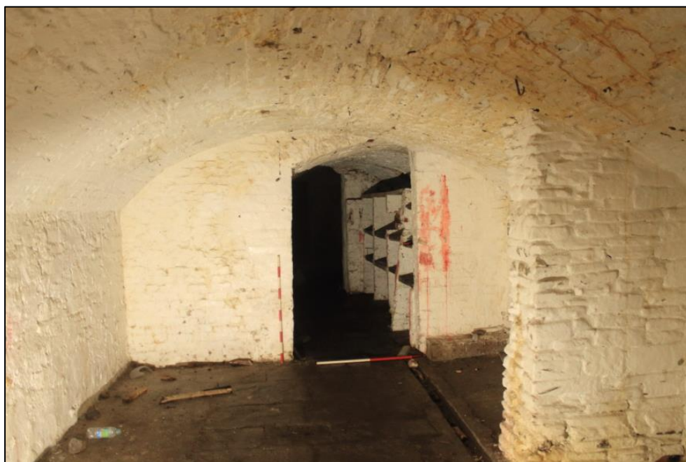
Photo 16: View south of Room 3 looking into Corridor 1. 1m scales.
