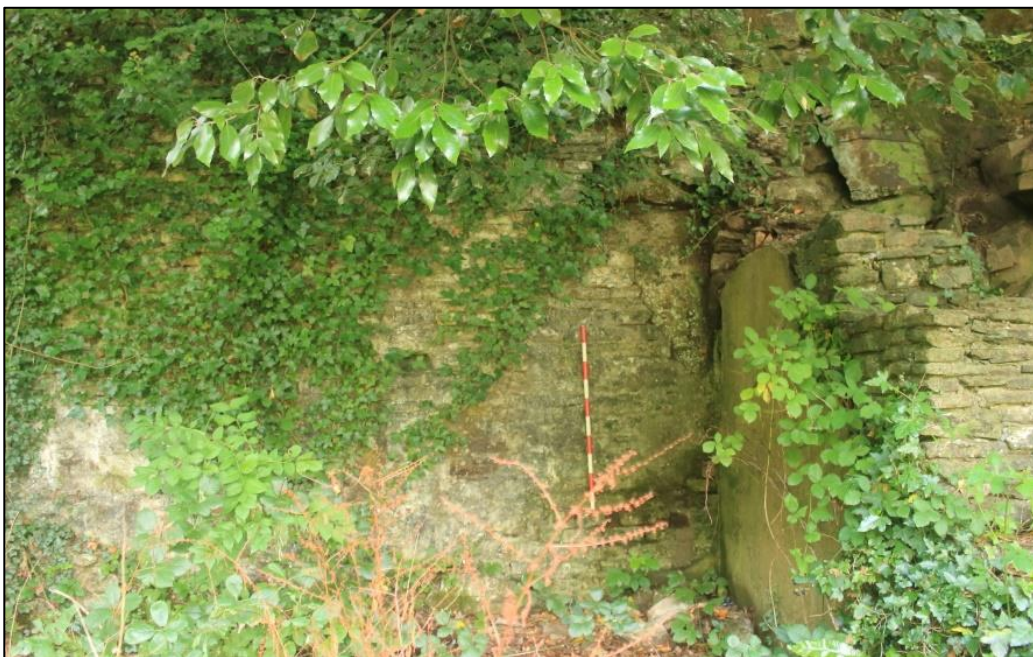
Photo 67: View east of the eastern wall of a detached room built against the quarried rock face. 1m scale.
