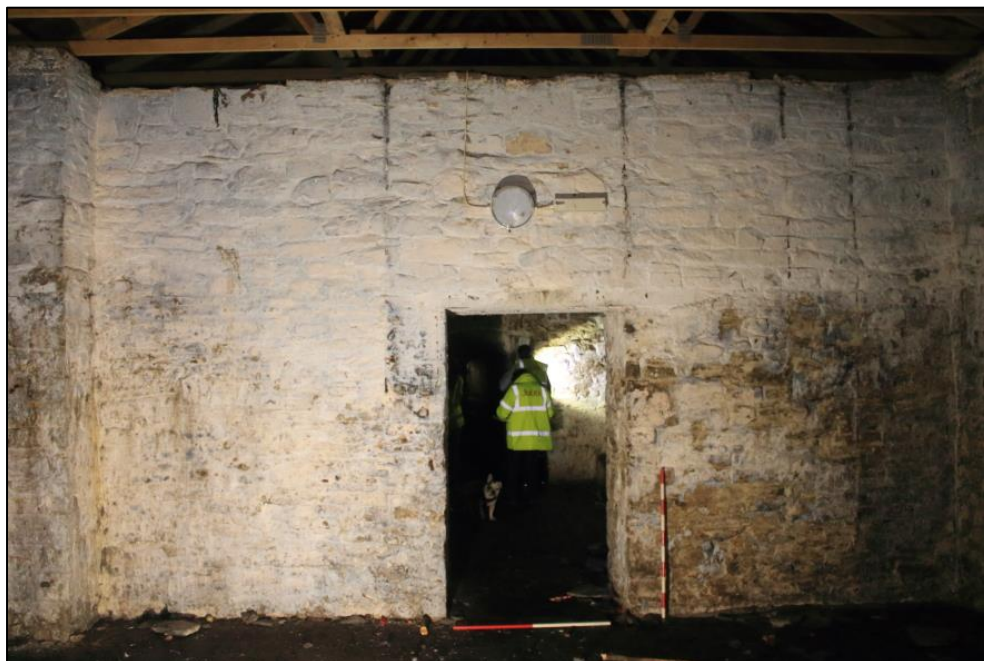
Photo 7: View north of north wall and doorway in Cellar Room 1. 1m scales.
