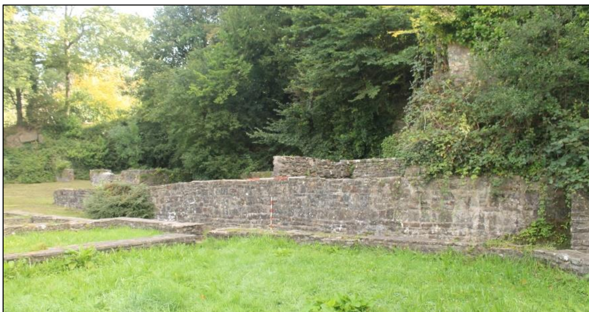
Photo 62: View northeast of retaining wall along the eastern side of Gnoll House. 2m and 1m scales.
