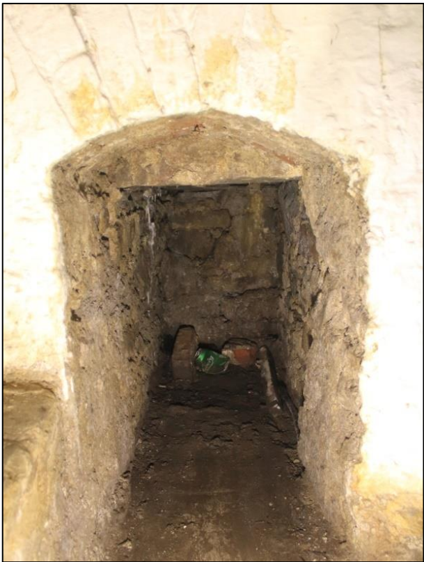
Photo 23: View west of the interior of the opening in the west wall of Room 4 (Compartment B).
