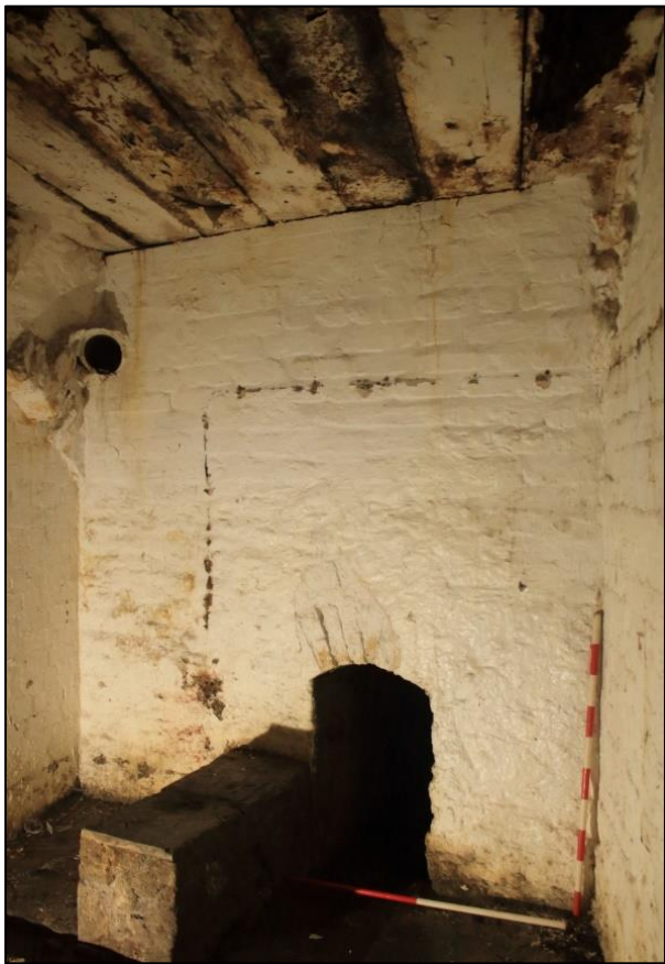
Photo 22: View west of the opening in the west wall of Room 4 (Compartment B). 1m scales.
