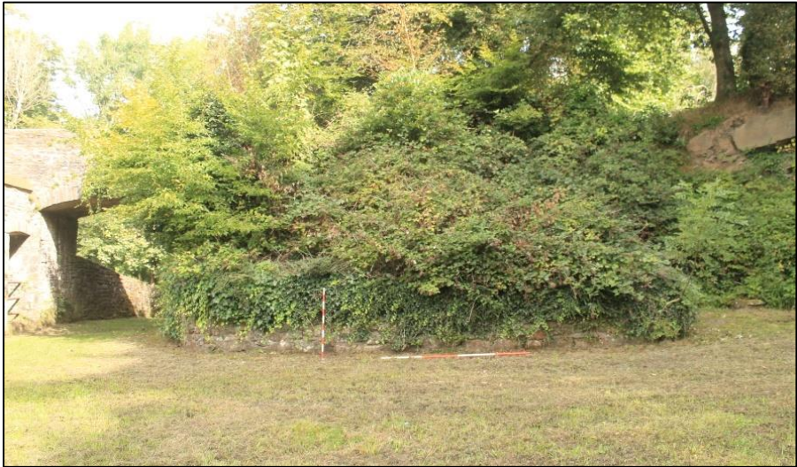
Photo 74: View north showing the retaining wall running up the entrance structure on the left. 2m and 1m scales.
