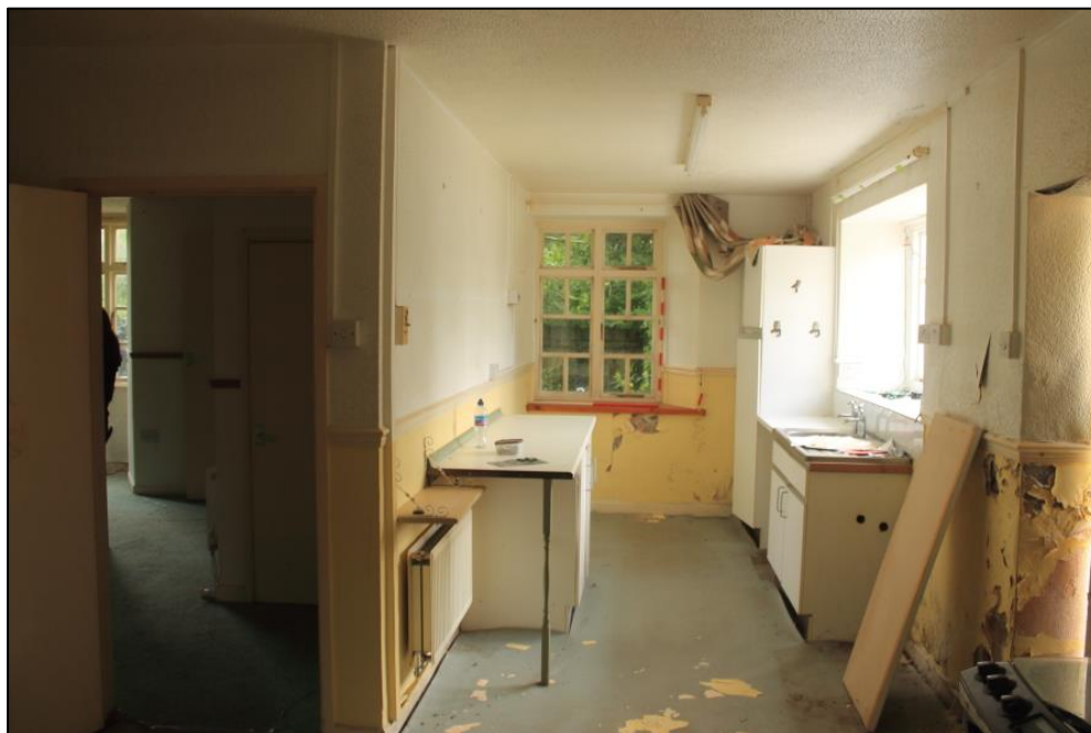
Photo 106: View east of the kitchen with doorway to the living room on the left. 1m scales.
