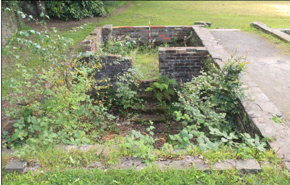
Photo 57: View south across the brick structure at the southeast end of Gnoll House. 2m and 1m scales.
