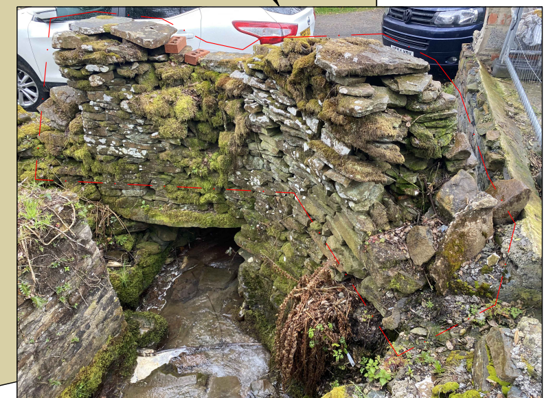
Area of wall to be removed and reinstated
